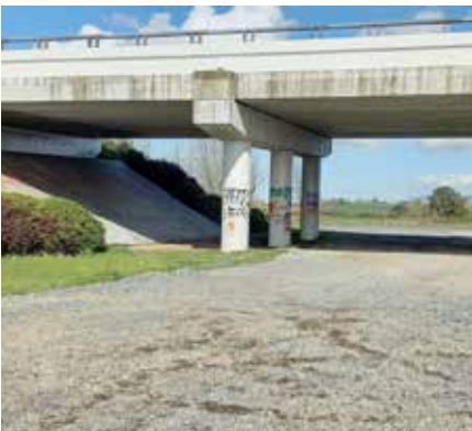
Chalmers Road underpass of Waikato Expressway
