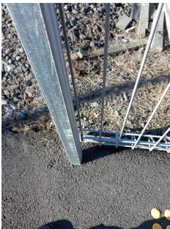
Figure 5-4. Minor damage to the pedestrian maze fence – rivet has broken.
