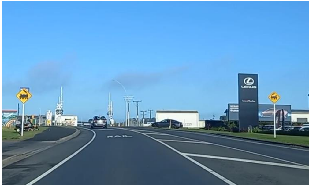
Figure 5-14. Advanced gated steam-train signs and RAIL-X road marking.
