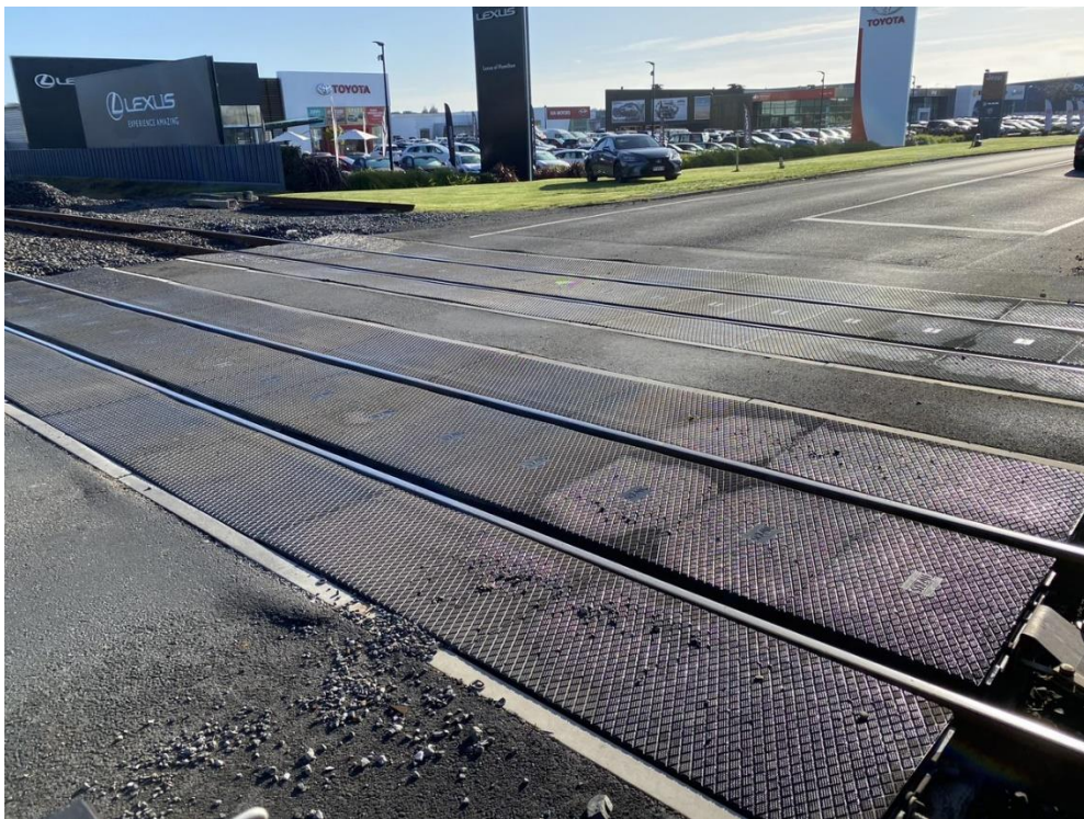
Figure 5-5. Debris and pooling water on the surface.
