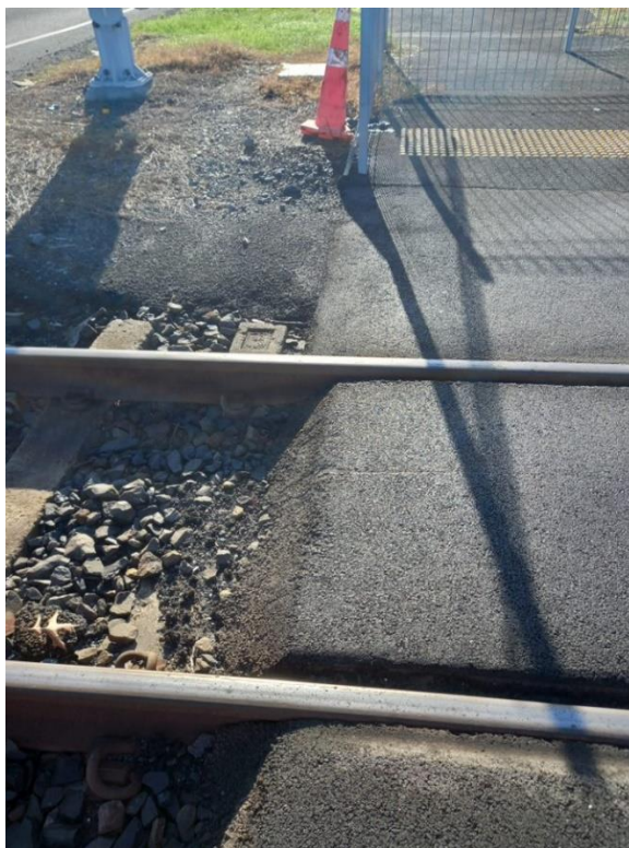
Figure 5-5. Pedestrian surface has flange gaps. The edge does not have tactile markings.
