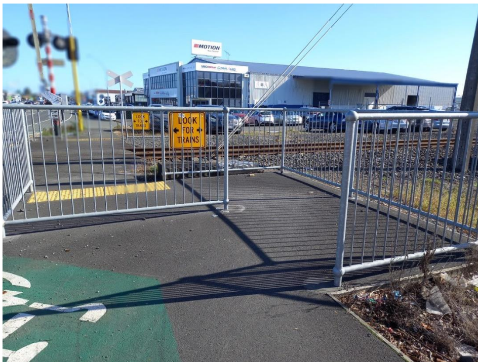
Figure 5-3. Te Kowhai Road pedestrian down crossing maze. West approach.
