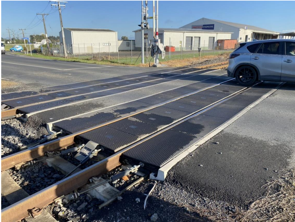
Figure 5-6. Road and Track Panel in good condition.
