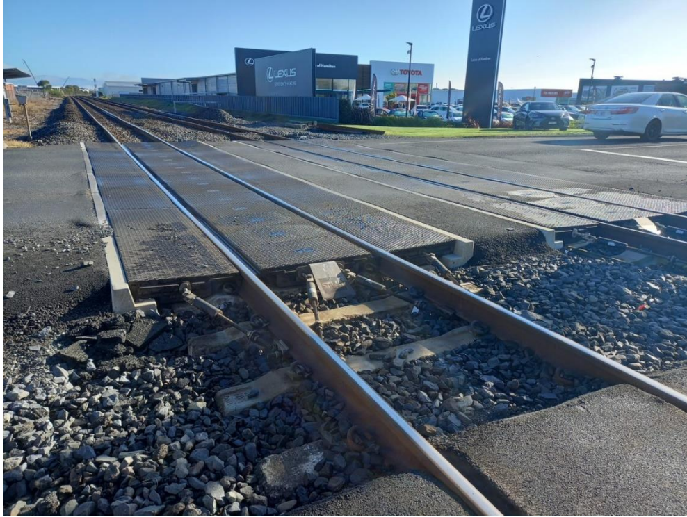
Figure 5-4. Te Kowhai Road level crossing surface dip is visible.
