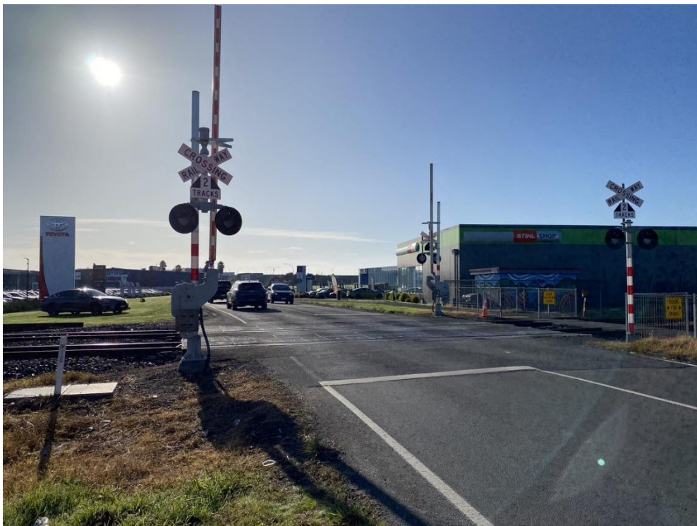
Figure 5-7. HAB and gated FLB from eastern approach.
