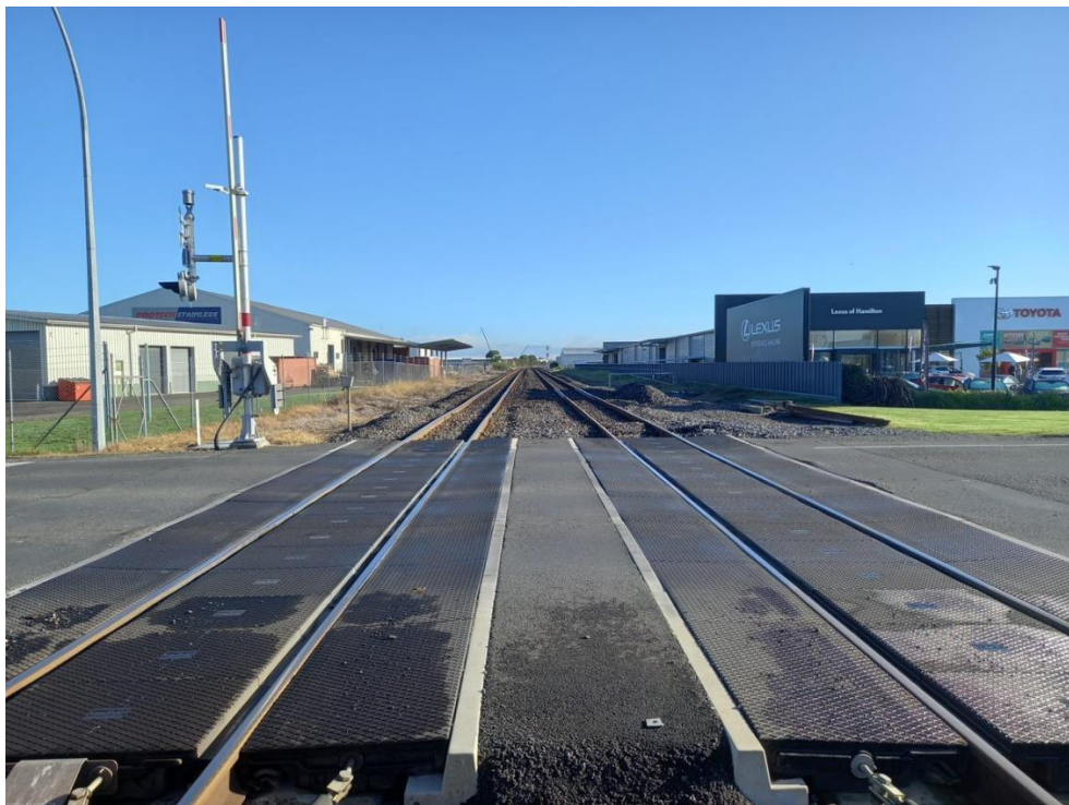
Figure 5-3. Te Kowhai Road level crossing surface.
