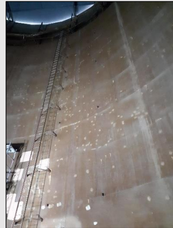
Figure 8 - 6 o'clock overview of spot corrosion on liner
