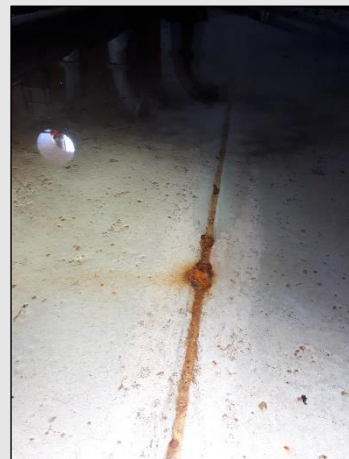
Figure 16 - Floor weld at panel 3 in from 6 o'clock
