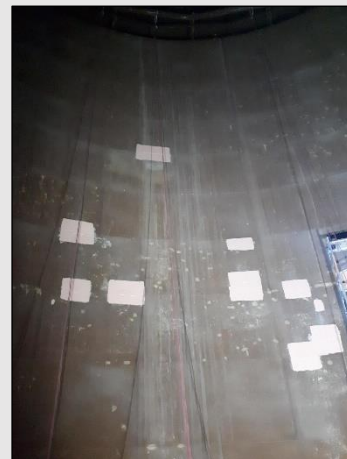
Figure 10 - 4 o'clock estimated surface area for repair at 25%
