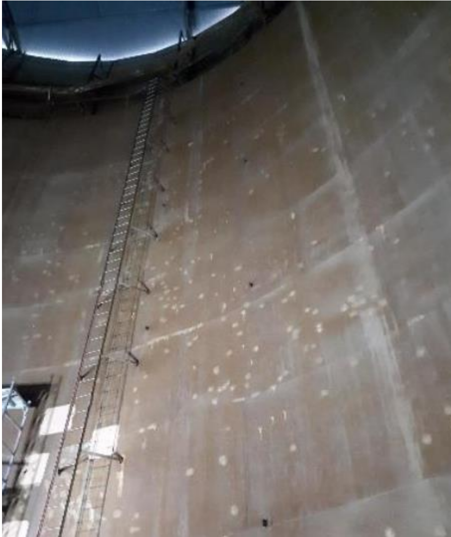
Figure 2-5. Overview of internal steel liner with spot corrosion (Altex Coatings, 2019)
