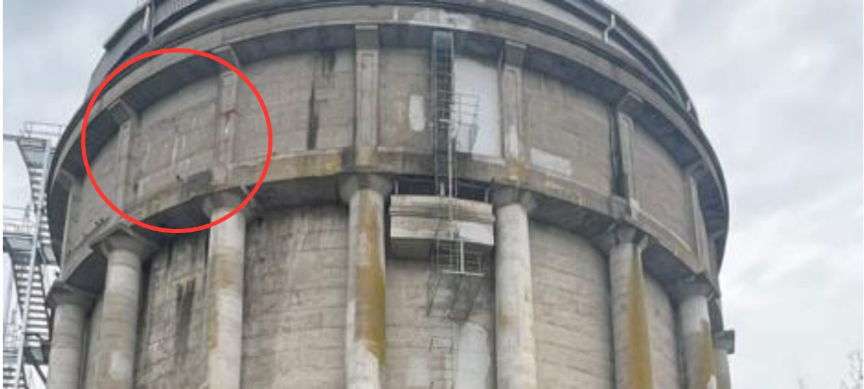
Figure 2-11. Evidence of leaking and reinforcement corrosion in the upper wall and rib (2025)
