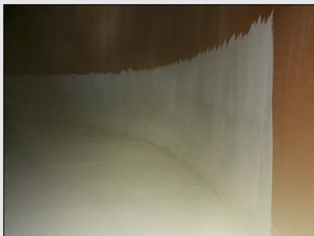
Figure 1 - 6-9 0'clock on wall to 2m roller coat applied coating DFT slightly less than existing
