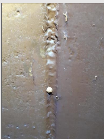
Figure 5 - Weld joint example with spot corrosion returned to power red oxide
