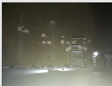
Figure 6 - Overview of patch repairs and corrosion cells looking at 3-6 o'clock worst area 2-7 o'clock corrosion pitting
