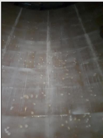
Figure 9 - 8 o'clock overview of spot corrosion on liner
