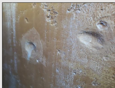
Figure 4 - Spot repairs on corrosion pitting about 4mm deep
