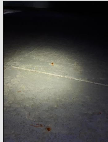
Figure 14 - Floor Spot corrosion at 4th panel in at 3 o'clock
