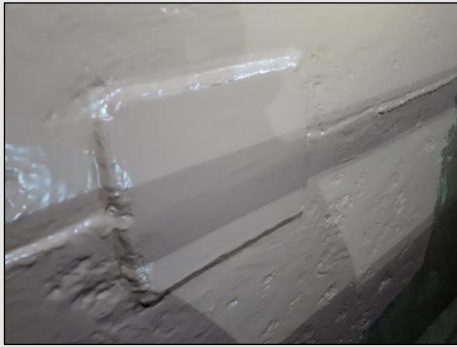
Figure 13 – Close up repair at 5 o'clock 3rd strake up full coating system
