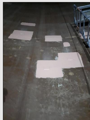
Figure 12 - New steel patch repairs welded and coated in Carboguard 504 and Altra~Shield 2000
