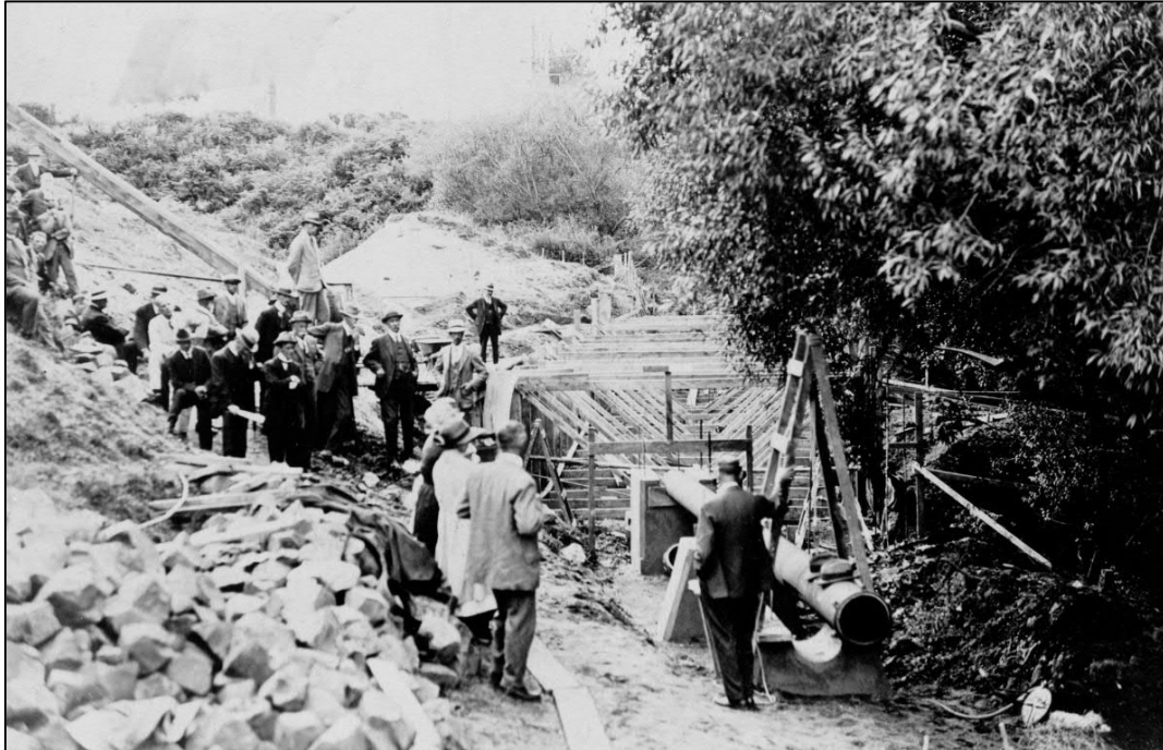
Figure 3: Hamilton waterworks - laying pipeline to reservoir (no date) (HCL_11584).
