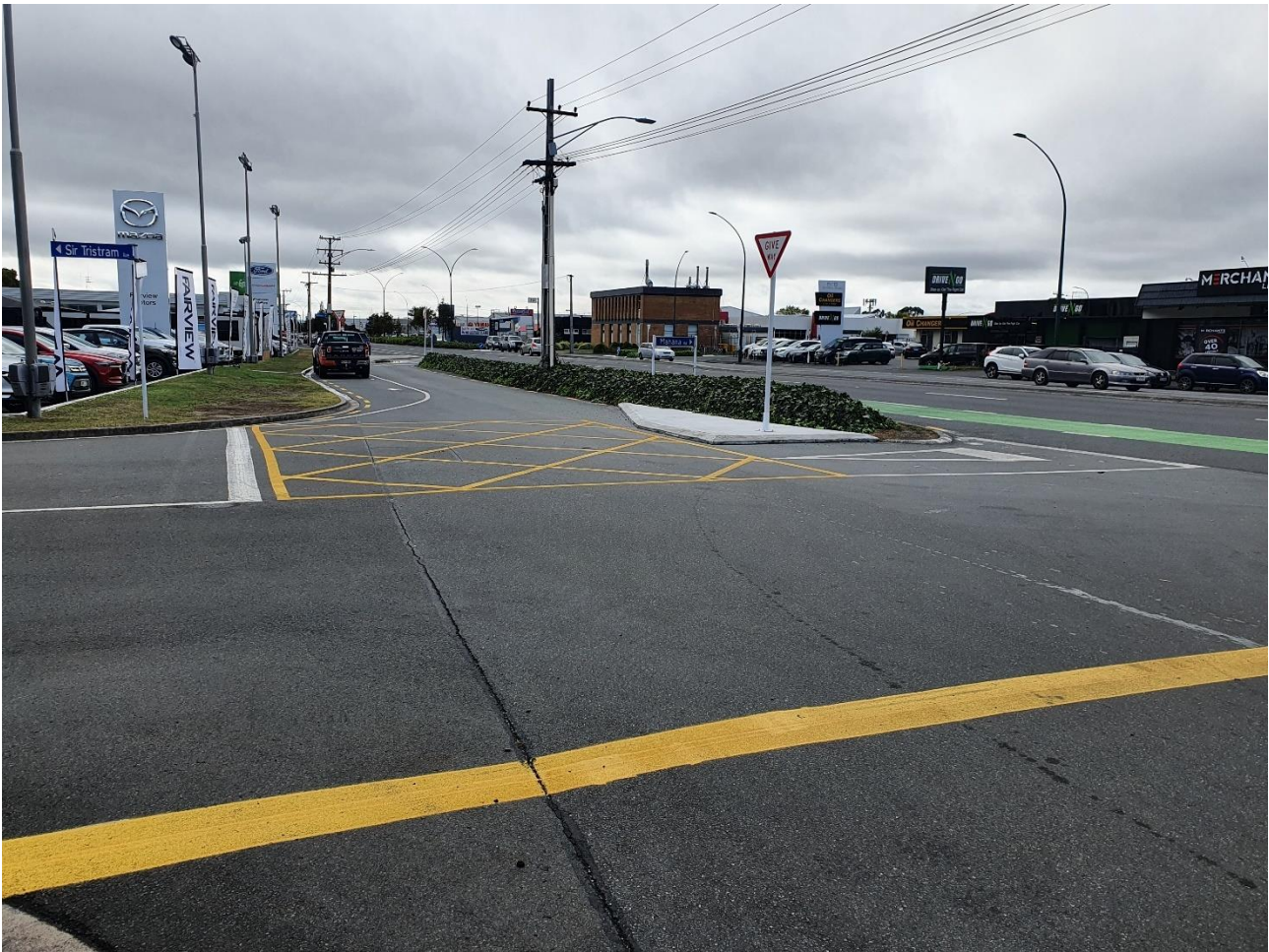
Figure 40: Te Rapa Road / Sir Tristram Avenue Intersection Layout after Construction
