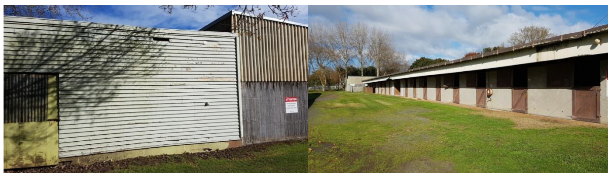
Figure 6. Typical existing horse stable construction at site showing painted timber (left) and concrete walls of individual stalls (right)
