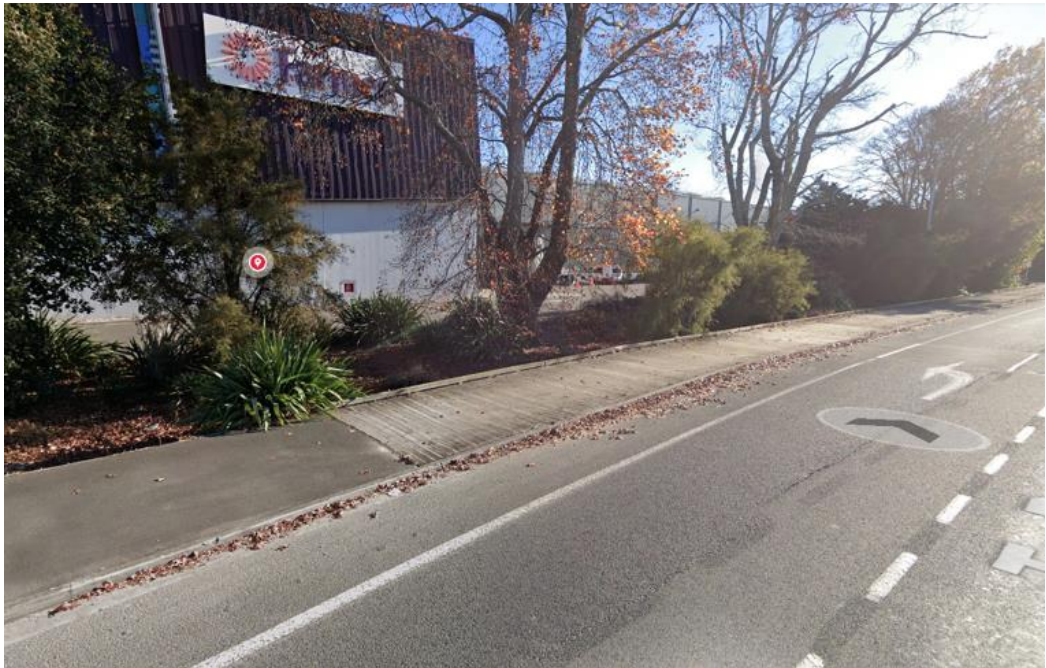
Figure 16: Existing Boardwalk adjacent to The Base on Te Rapa Road
