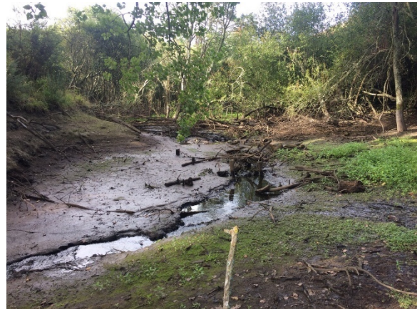
Figure 75: Watercourse upstream of the buried culvert MGK_E_Trib2_5.
