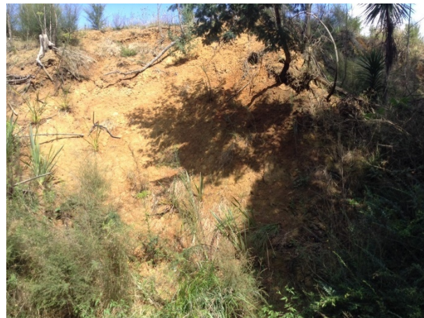
Figure 47: Erosion hotspot on true left bank MGK_W_Main_12 (Stan Heather development).
