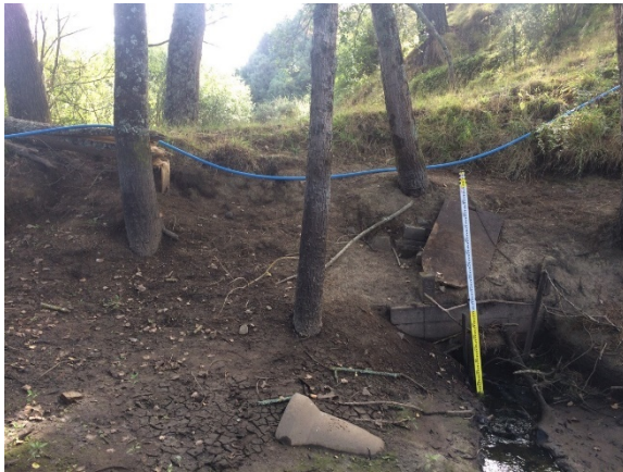
Figure 74: Buried culvert under farm crossing with wetland floodplain downstream.
