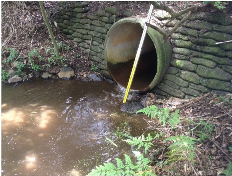
Figure 123: Fish barrier under John Webb Drive.
