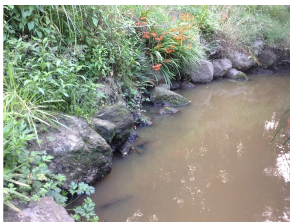
Figure 10: Toe protection at MGK_Main_5.
