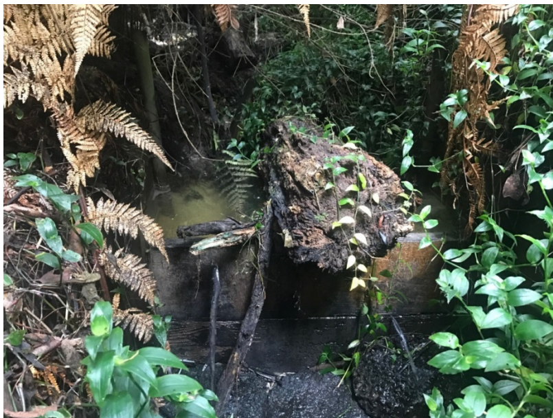
Figure 140: Wooden weir structures upstream of high erosion reach MGK_W_Trib3_1.
