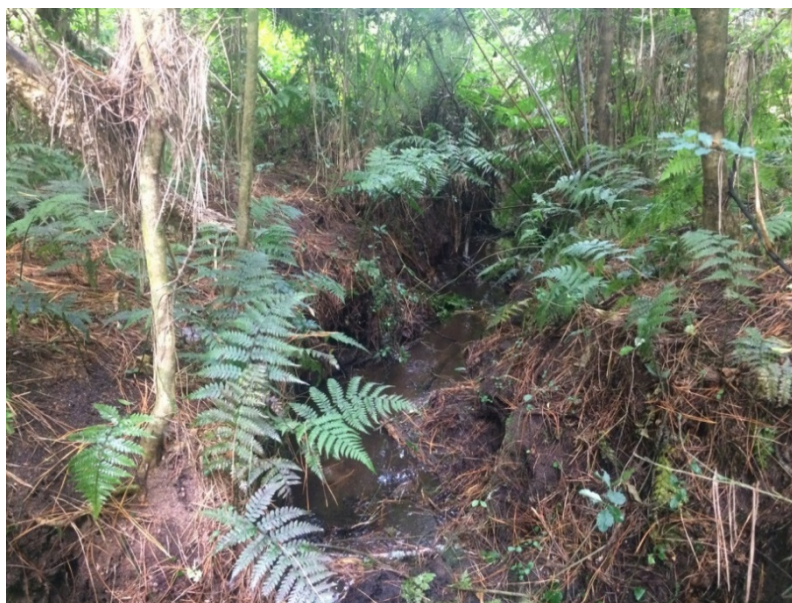
Figure 141: Erosion hotspot along MGK_E_Trib3_1.
