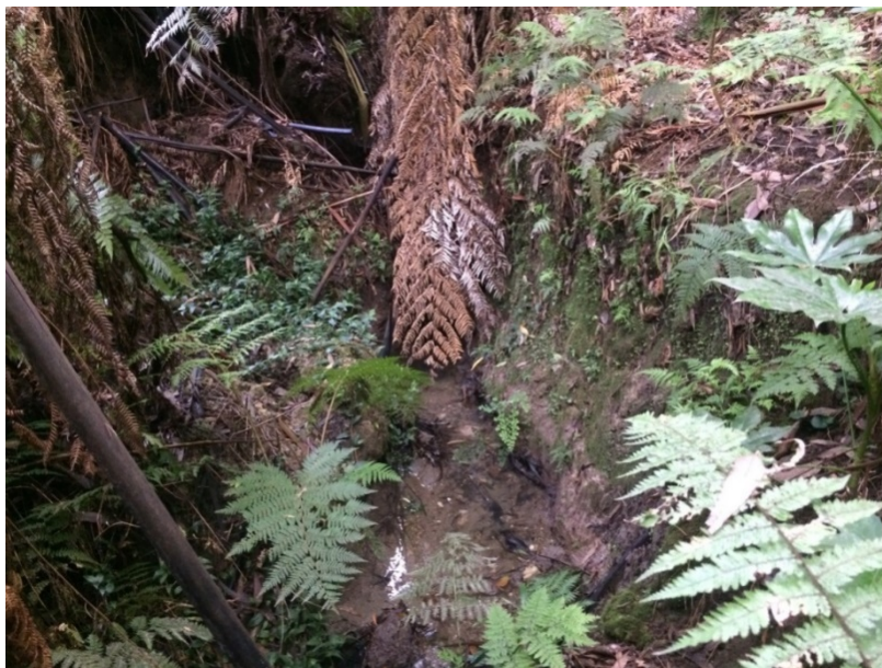
Figure 135: Incised reach at MGK_C_Trib4.
