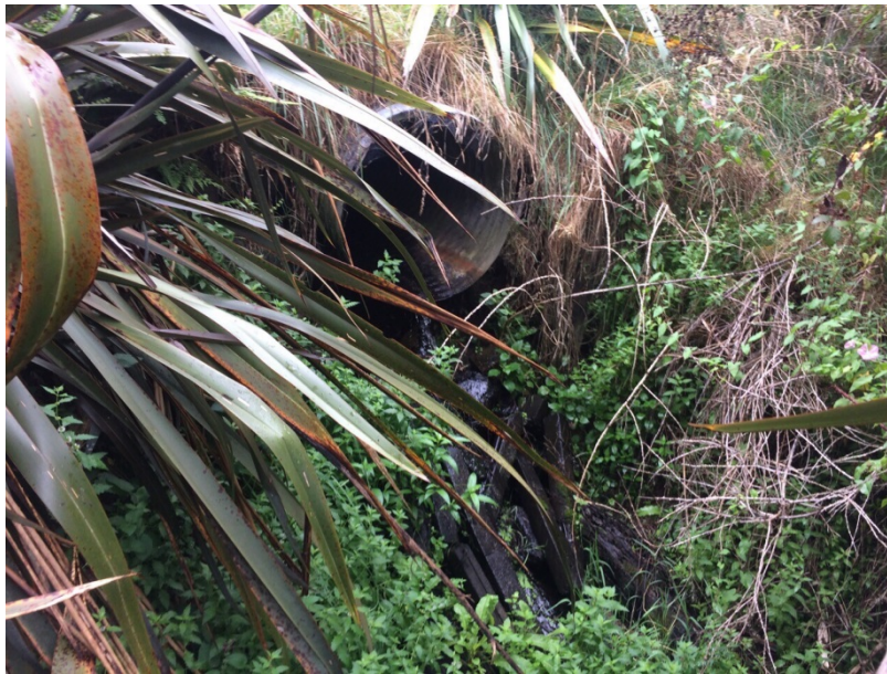
Figure 128: Spat rope fitted at culvert upstream of MGK_E_Trib6_1.
