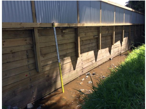
Figure 26: Timber bank lining along property at MGK_C_Fork1_2.
