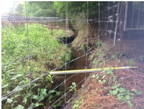
Figure 110: Channel along MGK_E_Main_17.
