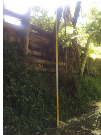
Figure 24: Bank lining above culvert at MGK_C_Fork1_1.
