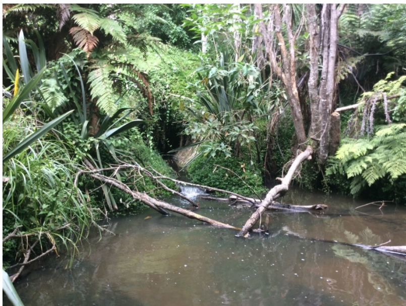
Figure 125: Outlet of Waterford Road culvert.
