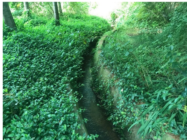
Figure 53: Concrete lined channel on MGK_W_Trib5_7.
