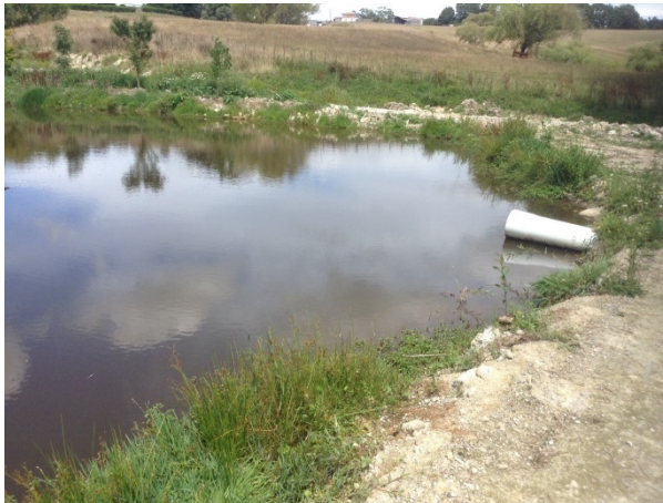
Figure 80: Eighth pond in series at 143 Hall Road recently constructed.
