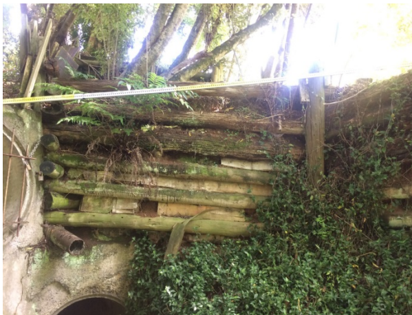
Figure 23: Bank lining above culvert at MGK_C_Fork1_1.
