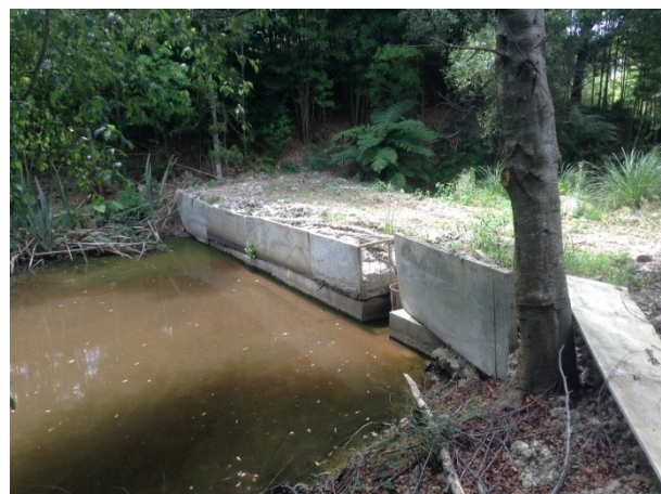
Figure 77: Concrete dam structure.
