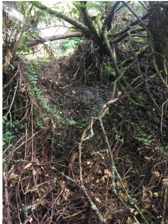
Figure 18: Landslip on true right bank on MGK_C_Trib1_1.
