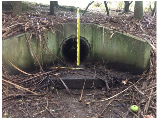
Figure 89: culvert under driveway of MGK_E_Trib3_6.
