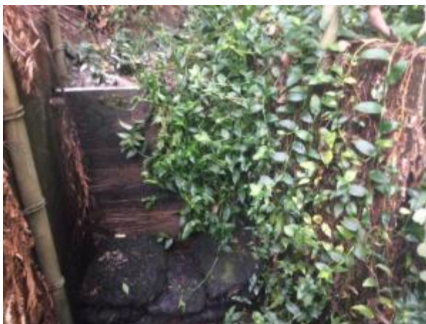
Figure 45: Timber weir along MGK_W_Trib3.
