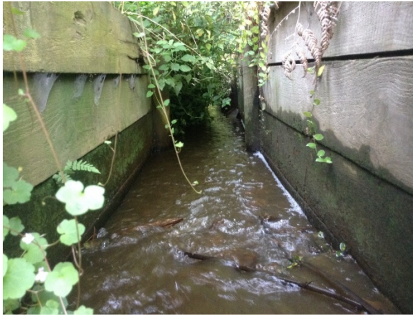
Figure 25: Bank lining extending 40 m at MGK_C_Fork1_2.
