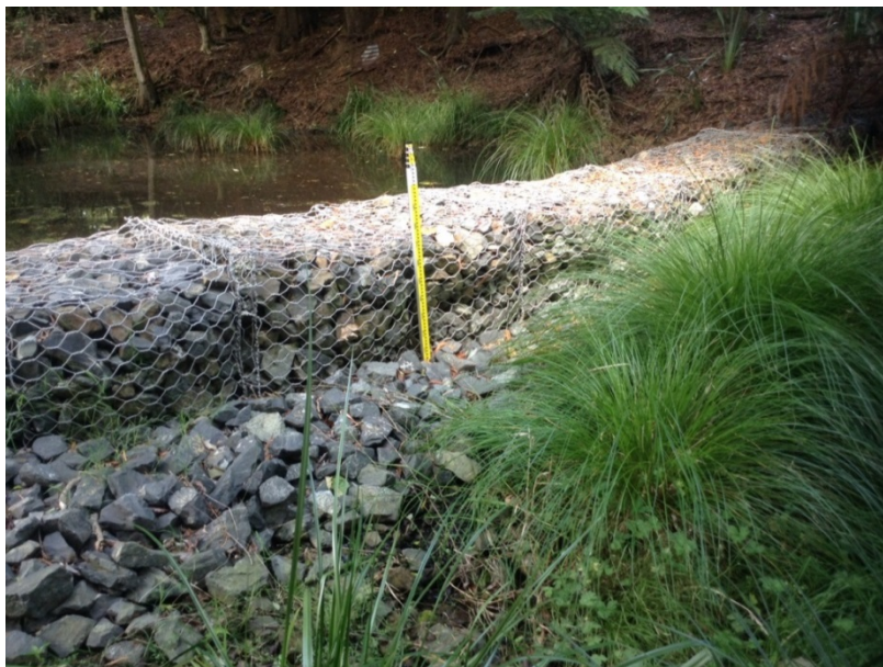
Figure 124: Carbourne Wetlands fish barrier.
