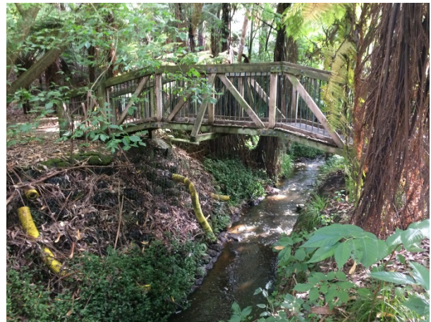
Figure 16: Bank lining along MGK_C_Main_4.
