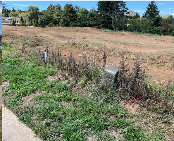
Figure 7: Services in place for 4 x Sections
