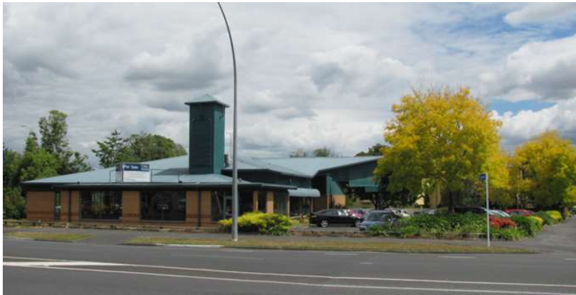
Figure 1.4.5b: Existing situation on Key Development Site 1 (2014)
