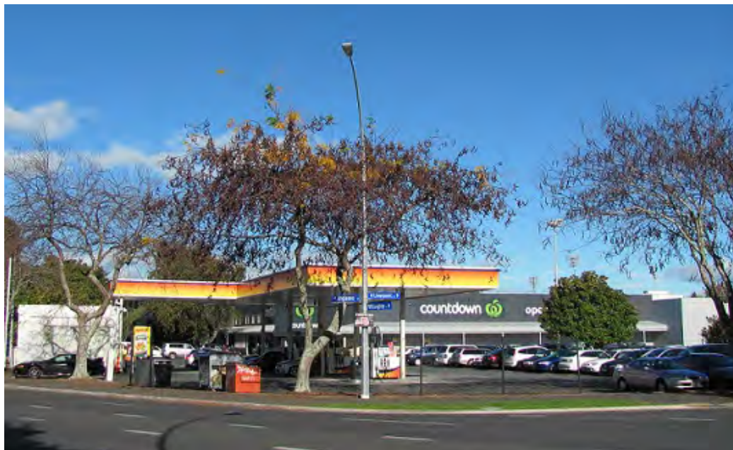
Figure 1.4.5mm: Existing situation on Key Development Site 5 (2014)
