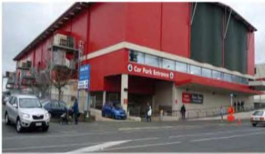
Figure 1.4.5ee: Existing situation on Key Development Site 4 (2011)
