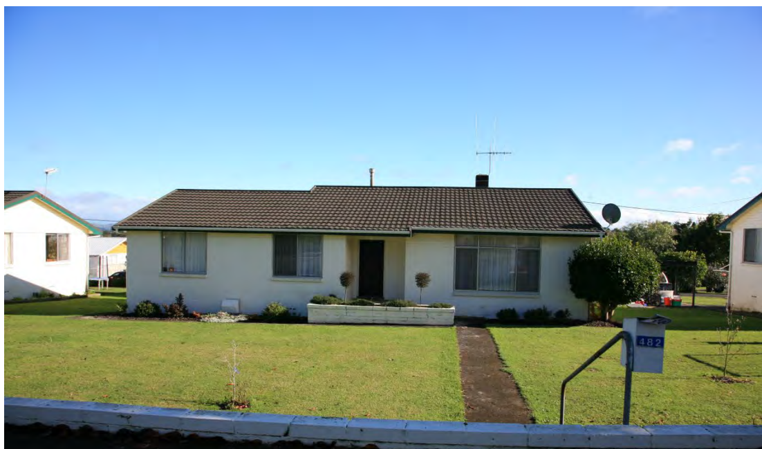
Figure 1.4.9k: 2012 photograph showing the typology of the original Teacher Housing on Tuhikaramea Road
