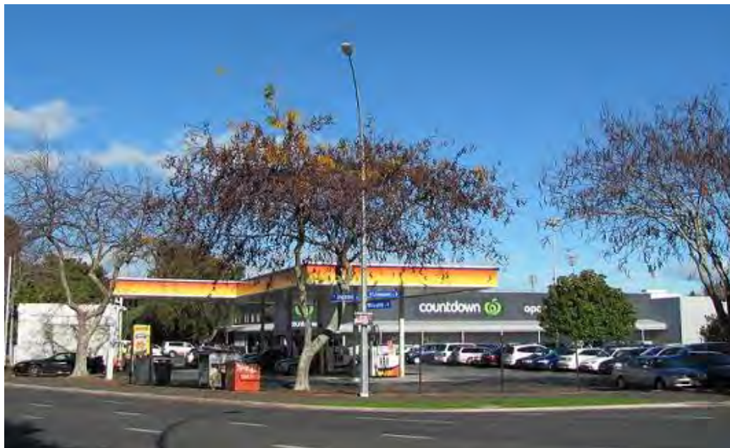
Figure 1.4.5mm: Existing situation on Key Development Site 5 (2014)
