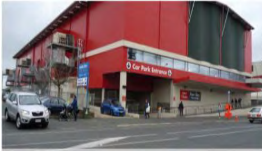
Figure 1.4.5ee: Existing situation on Key Development Site 4 (2011)
