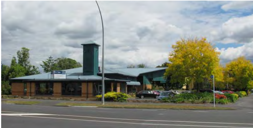
Figure 1.4.5b: Existing situation on Key Development Site 1 (2014)
