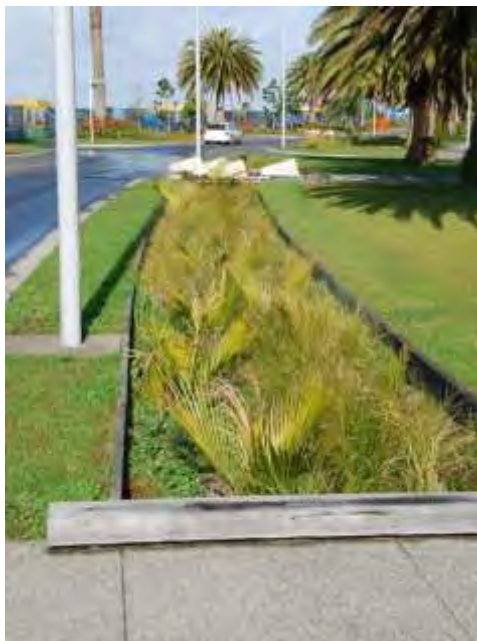
Figures 1.4.2h and i: Examples of swales to manage stormwater (from Hobsonville and Long Bay, Auckland)
