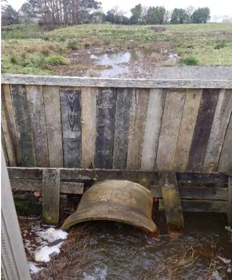
Culvert requiring remediation upstream of pond
