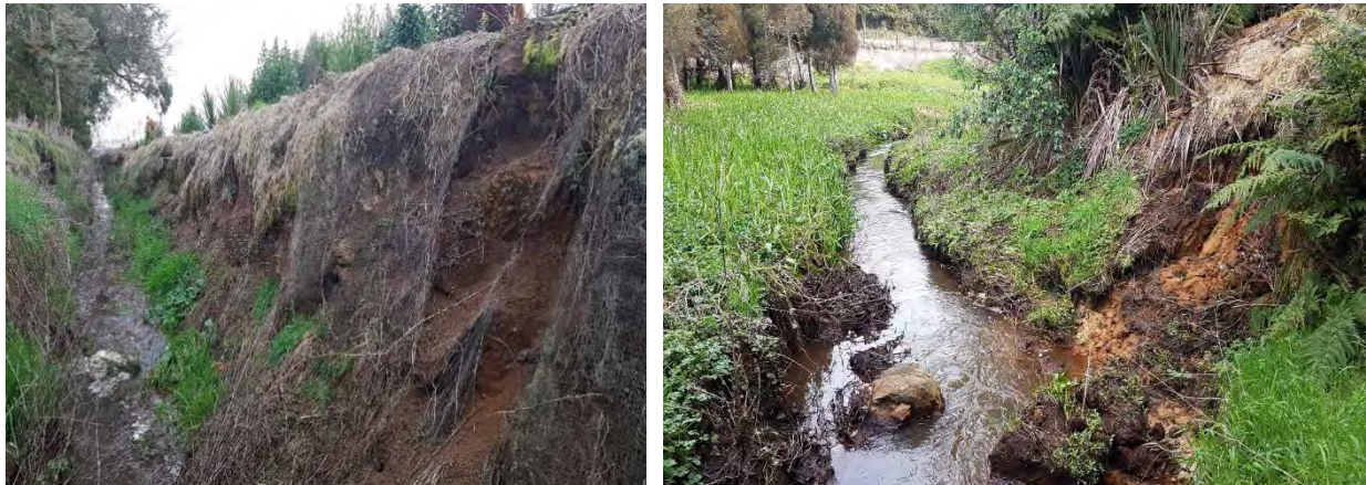
Figure 10: Left: Erosion and coir lining on banks upstream of the Te Kowhai Road culvert (UNK031); Right: Erosion downstream of outlet UNK107
