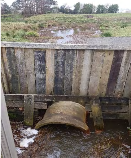
Culvert requiring remediation upstream of pond
