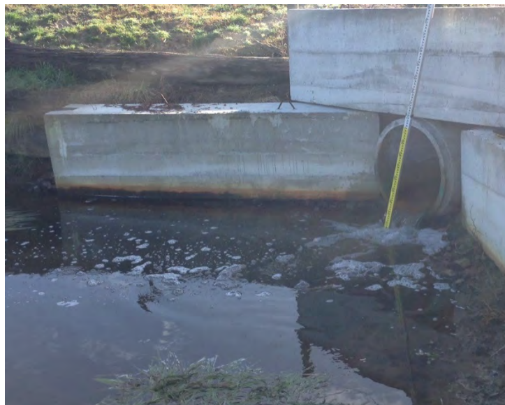
Figure 9: Fish barrier for swimming fish species located on the culvert outlet (Asset ID: UNK026)
