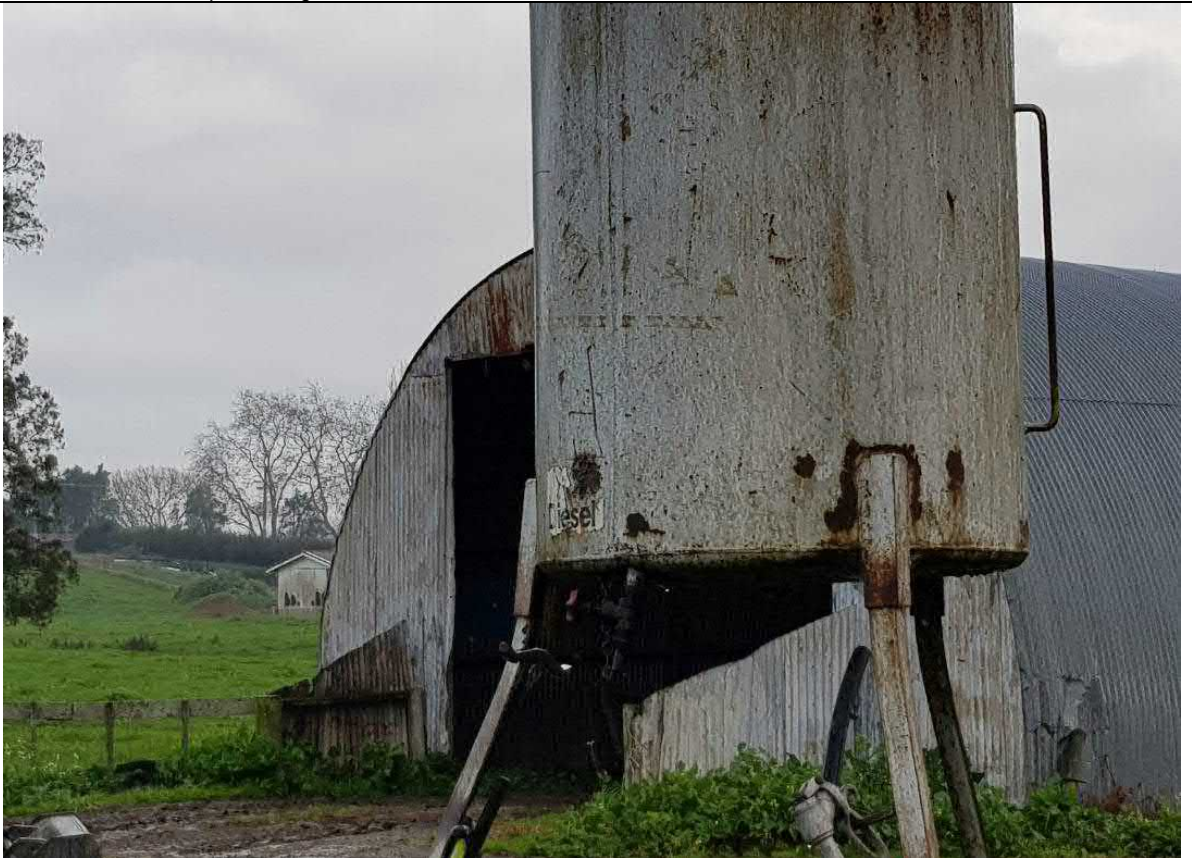
Photo 16. Standing diesel tank, facing south-west. PT LOT 7 DPS 15255.
