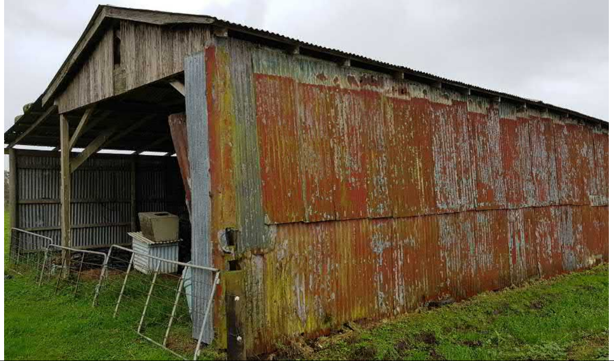
Photo 12. Storage shed, facing south-east. LOT 2 DP 485743.
