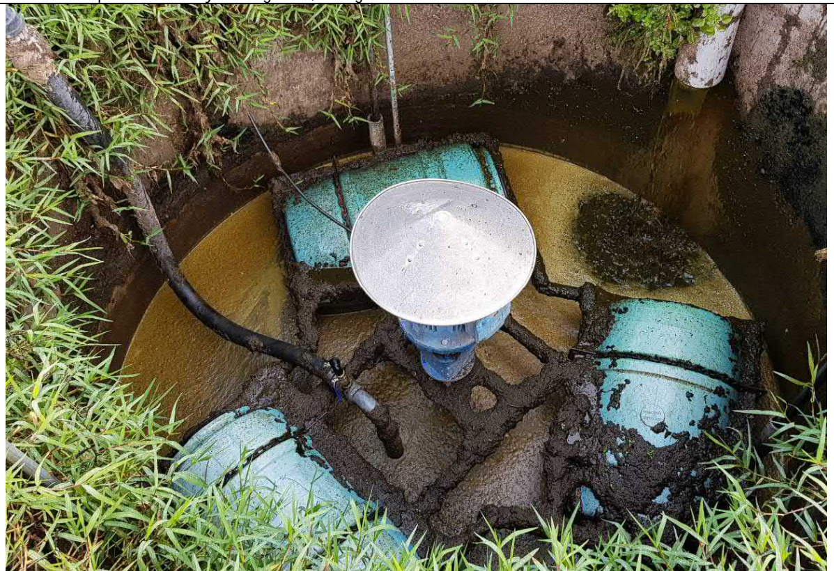
Photo 18. Effluent sump, connected to milking shed. PT LOT 7 DPS 15255.
