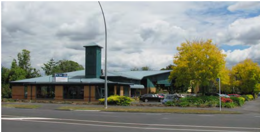
Figure 1.4.5b: Existing situation on Key Development Site 1 (2014)
