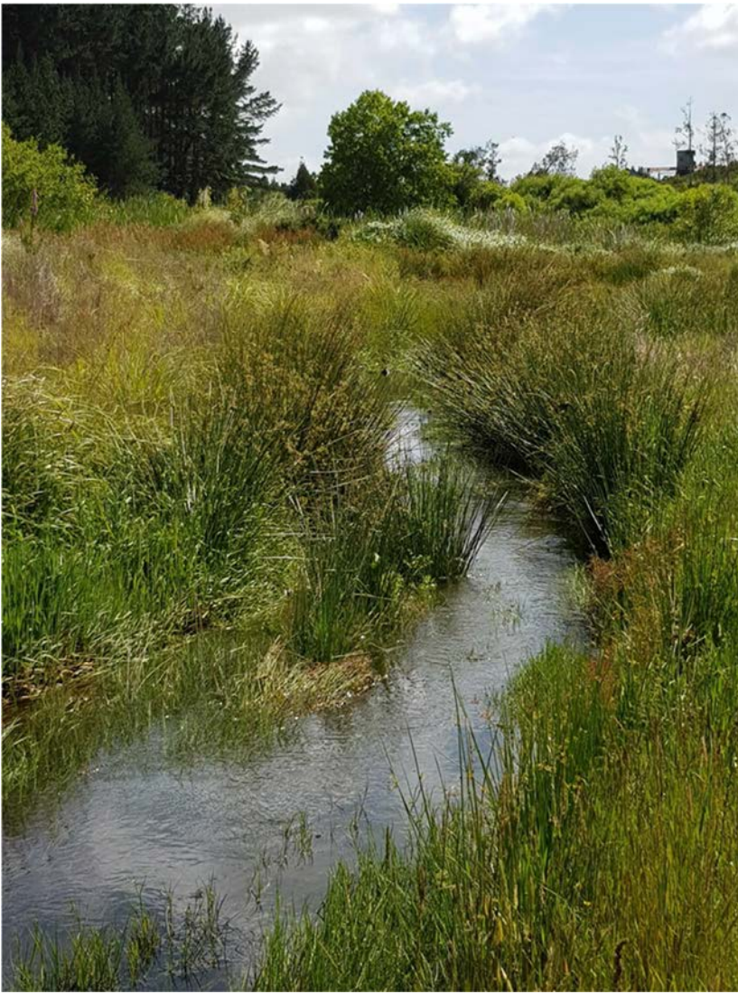
Figure 4-3 Example engineered stream and shallow floodplain. The stream has a low sinuosity and subtle bed apex geometry in the cross-section.
