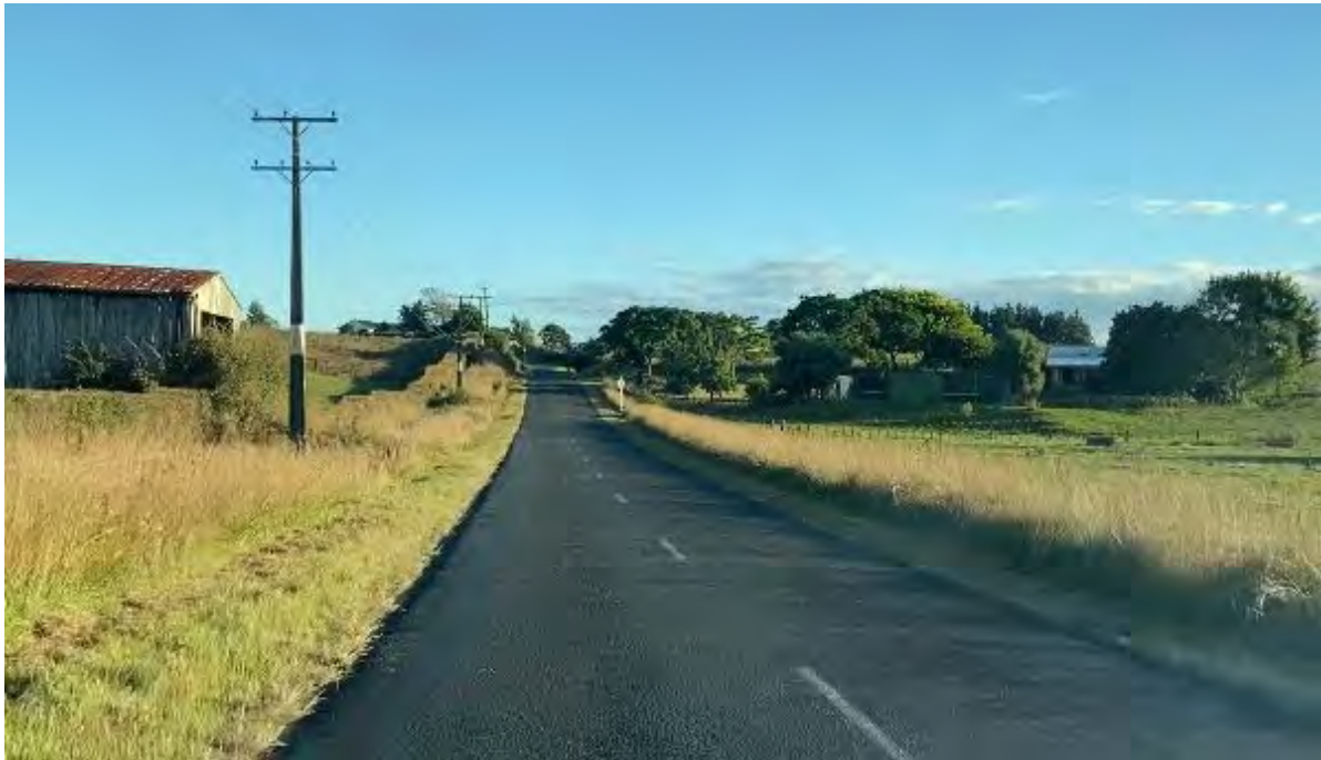
Photograph 2: Burbush Road – typical layout looking south
