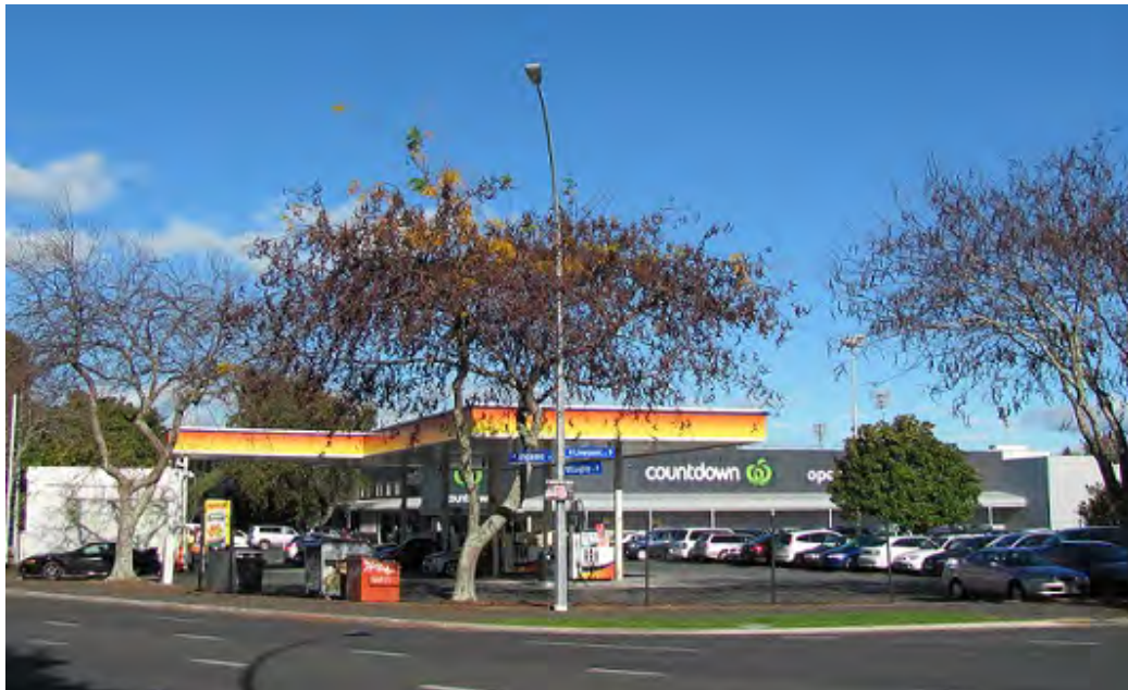
Figure 1.4.5mm: Existing situation on Key Development Site 5 (2014)
