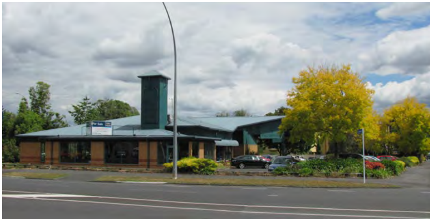
Figure 1.4.5b: Existing situation on Key Development Site 1 (2014)
