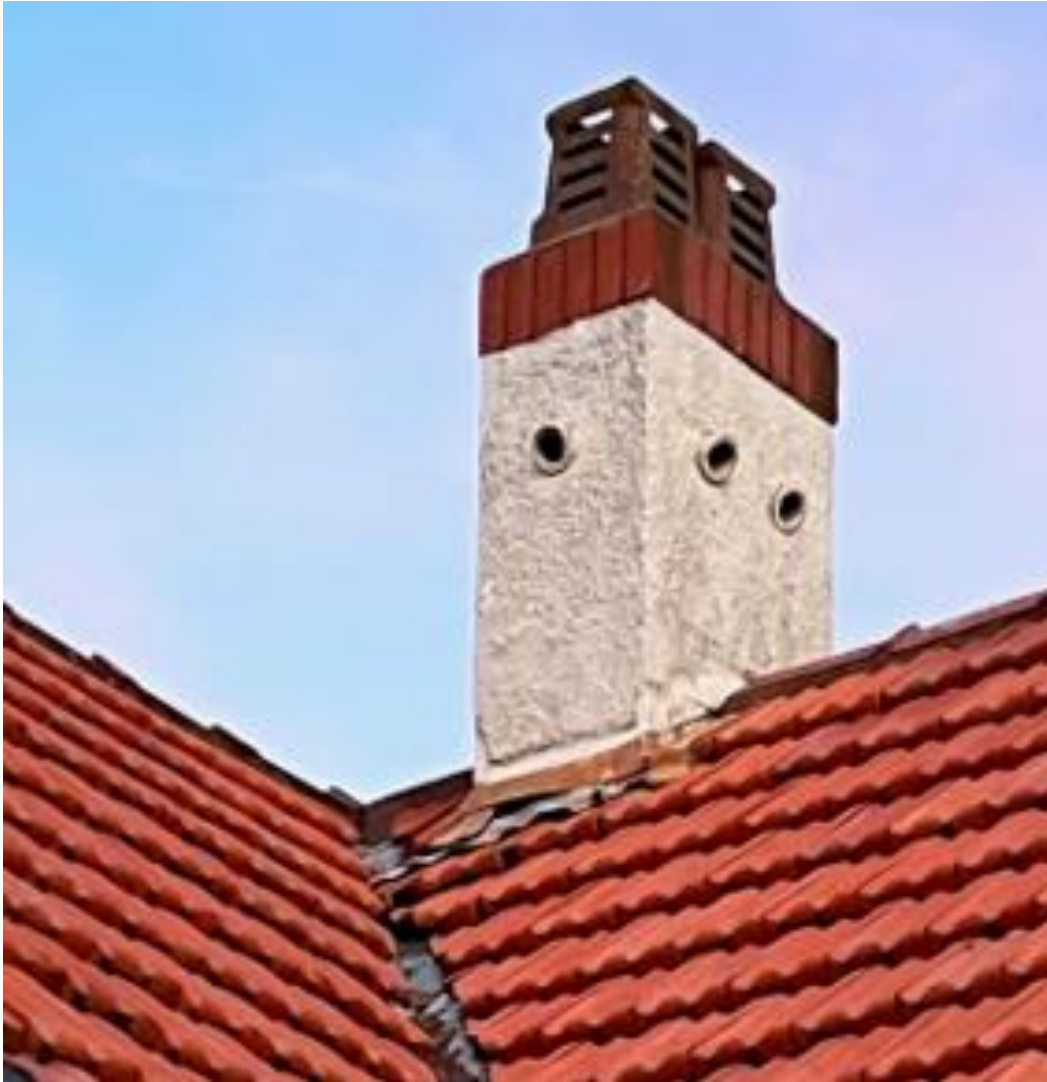
The tiles immediately below the chimney have slipped and exposed areas cause leaks. Also visible is corrosion in the guttering.
