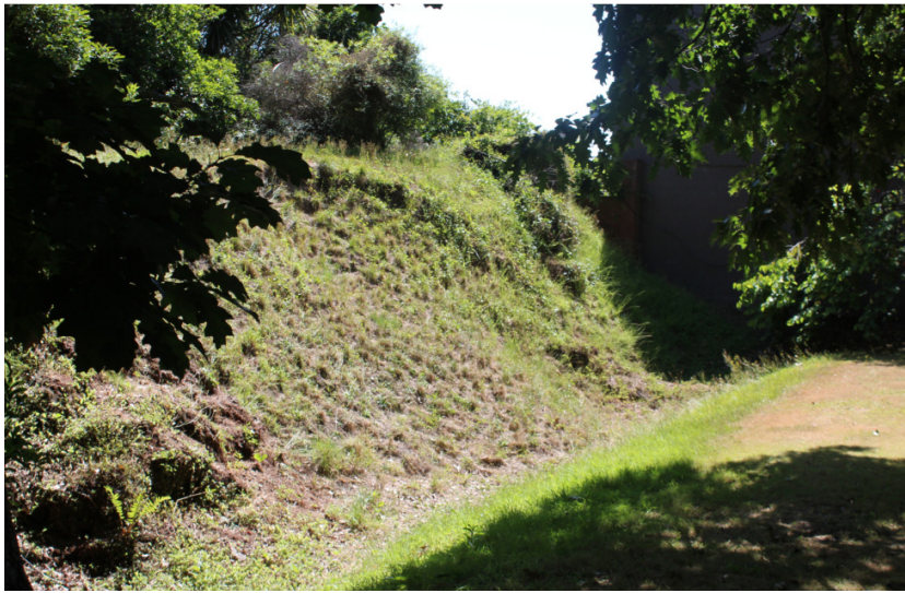
Figure 6. View of intact ditch defence at Miropiko Park, 31/01/2020.
