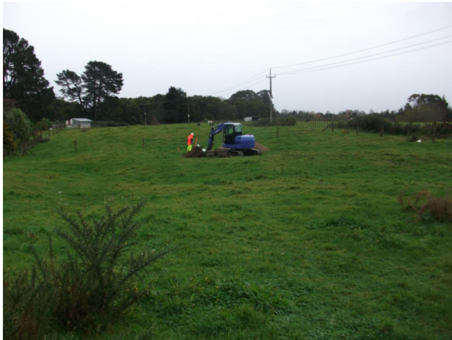
Figure 1. 2011 photograph of site S14/243 during geotechnical investigations. (Source: N. Cable).
