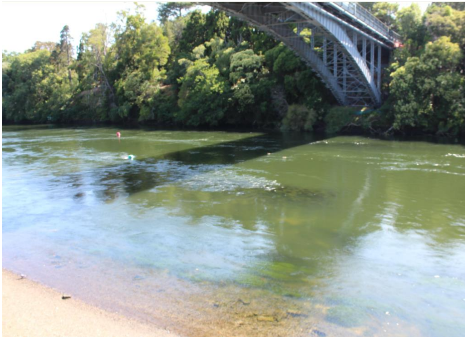
Figure 1. Remains of Union Bridge (S14/220) below Victoria Bridge, taken 31/01/2020.
