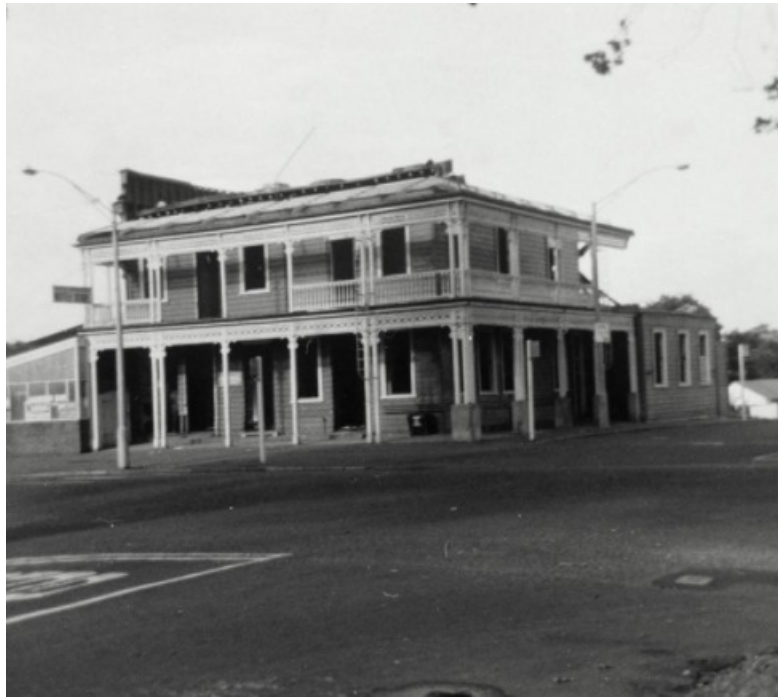
Figure 4. 1971 photograph of the Royal Hotel being demolished (source: Hamilton City Libraries Heritage Collection – HCL_14910 https://heritage.hamiltonlibraries.co.nz/objects/14910/royal-hotel-being-demolished ).
