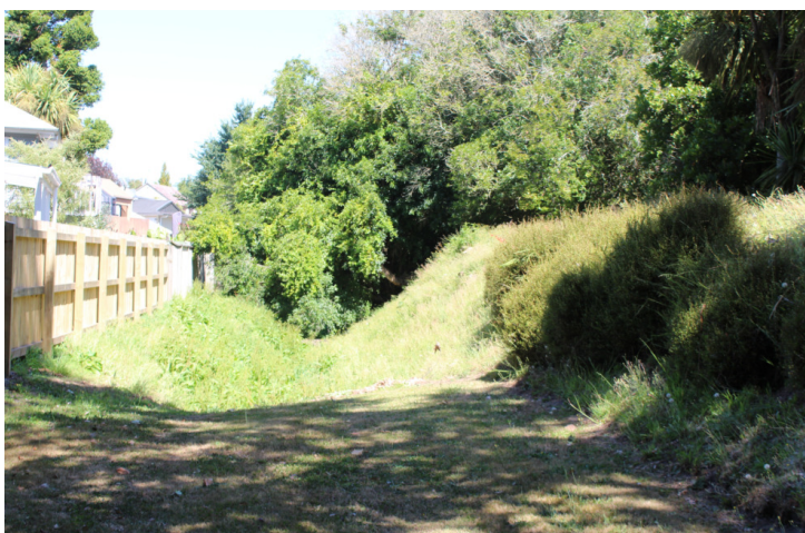
Figure 5. View of intact ditch defence at Miropiko Park, 31/01/2020.
