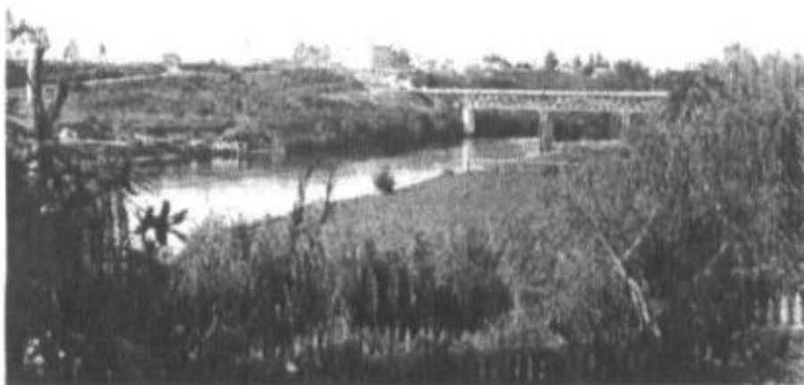
Figure 2: c.1890s view of the Union Bridge (ATL 1/1-001355-G) (Site Record Form).
