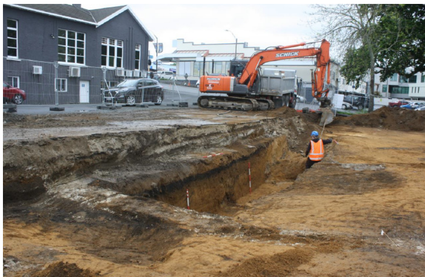
Figure 3: Image of trench excavated through Feature HV141 looking south. Reproduced from Keith 2021b: Figure 5 and including on the Site Record Form.
