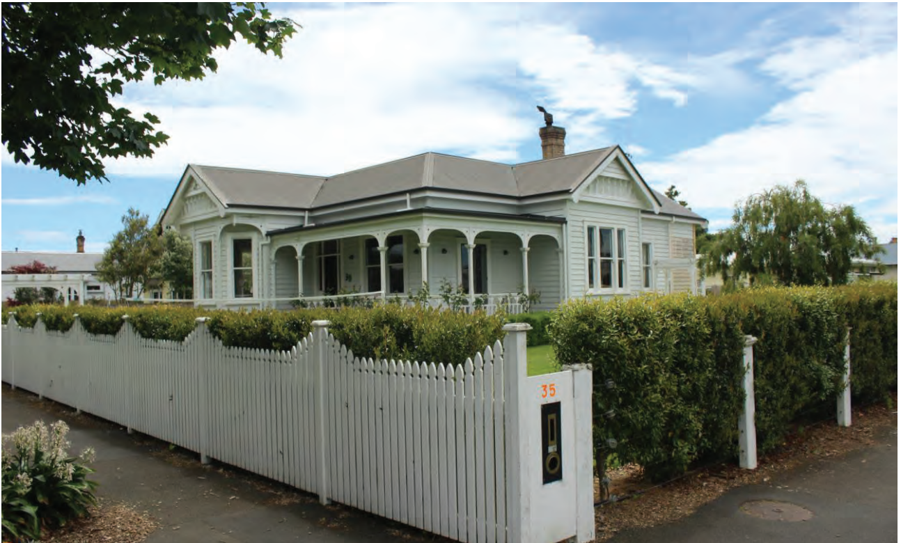
Figure 1: Villa at 35 Naylor Street.
