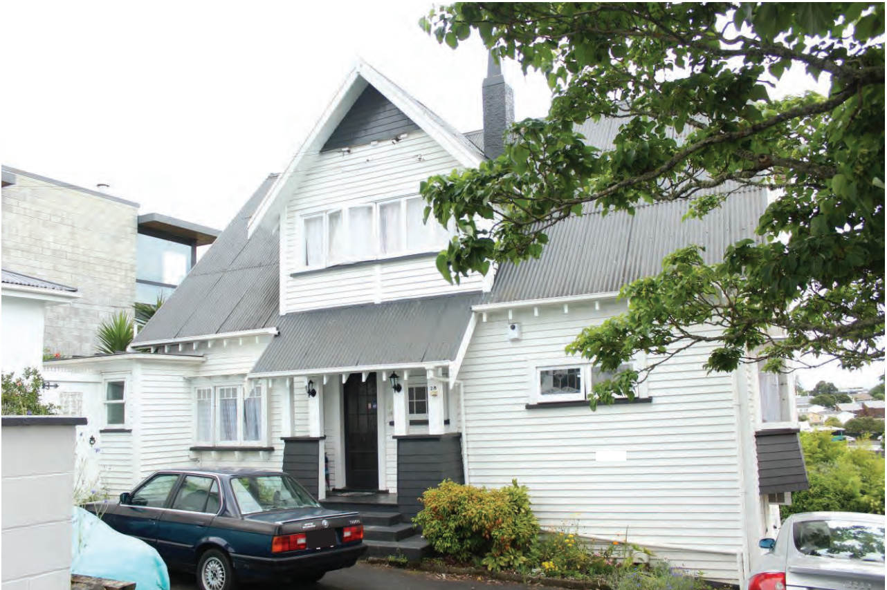
Figure 1: The building at 28 Thackeray Street.
