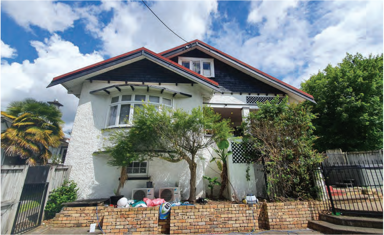
Figure 1: The dwelling at 31 Palmerston Street.
