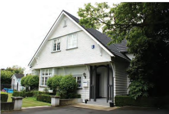
Figure 12: Arts and Crafts features of the building include a two-storey structure with an overhanging first storey and steeply pitched roof.
