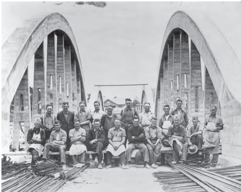
Figure 4: Construction workers on the Fairfield Bridge, c.1936. Source: Waikato Library Archives
