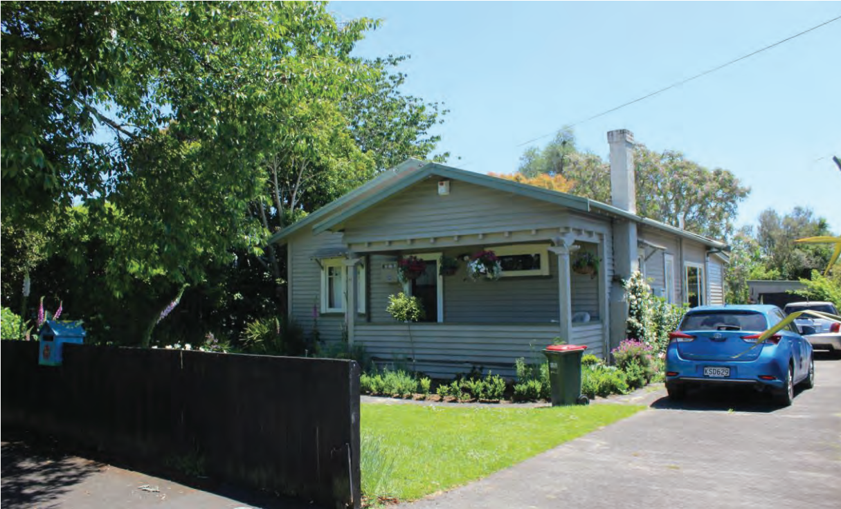
Figure 1: Bungalow at 17 Oxford Street.
