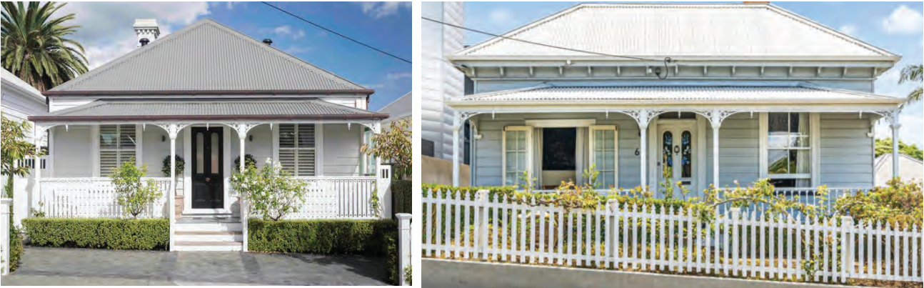
Figure 7 - Examples of 'early' or 'square' villas, built between 1880-1900. Source: Various
