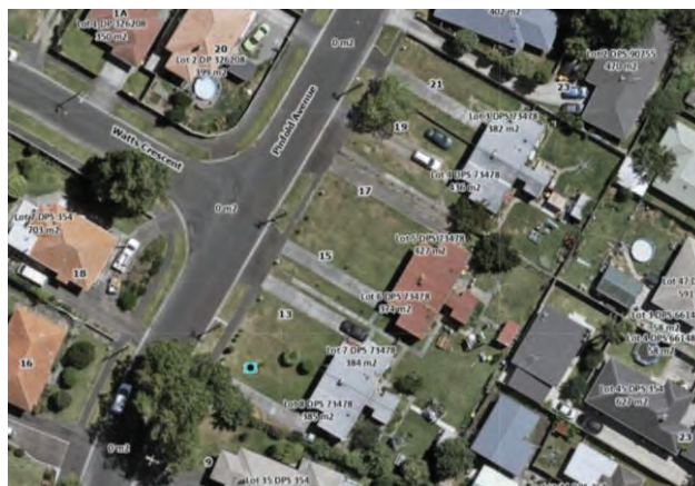
Figure 9: Aerial view of the three duplex flats. Source: HCC Aerials.
