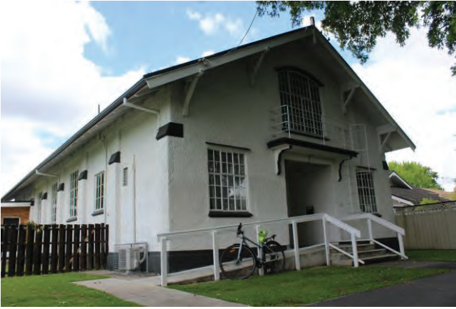
Figure 6: The hall at 24 Thames Street.
