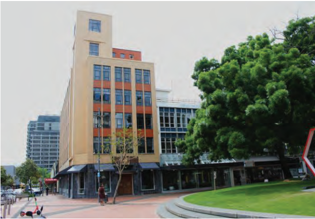
Figure 12: The Garden Place façade of the building.
