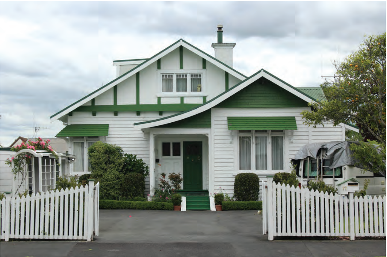
Figure 1: Dwelling at 17 Beale Street, 2021.
