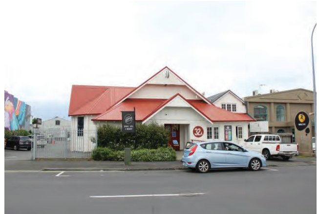
Figure 7: South (front) elevation as seen from the street.
