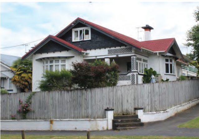
Figure 7: 31 Palmerston Street as viewed from the street.
