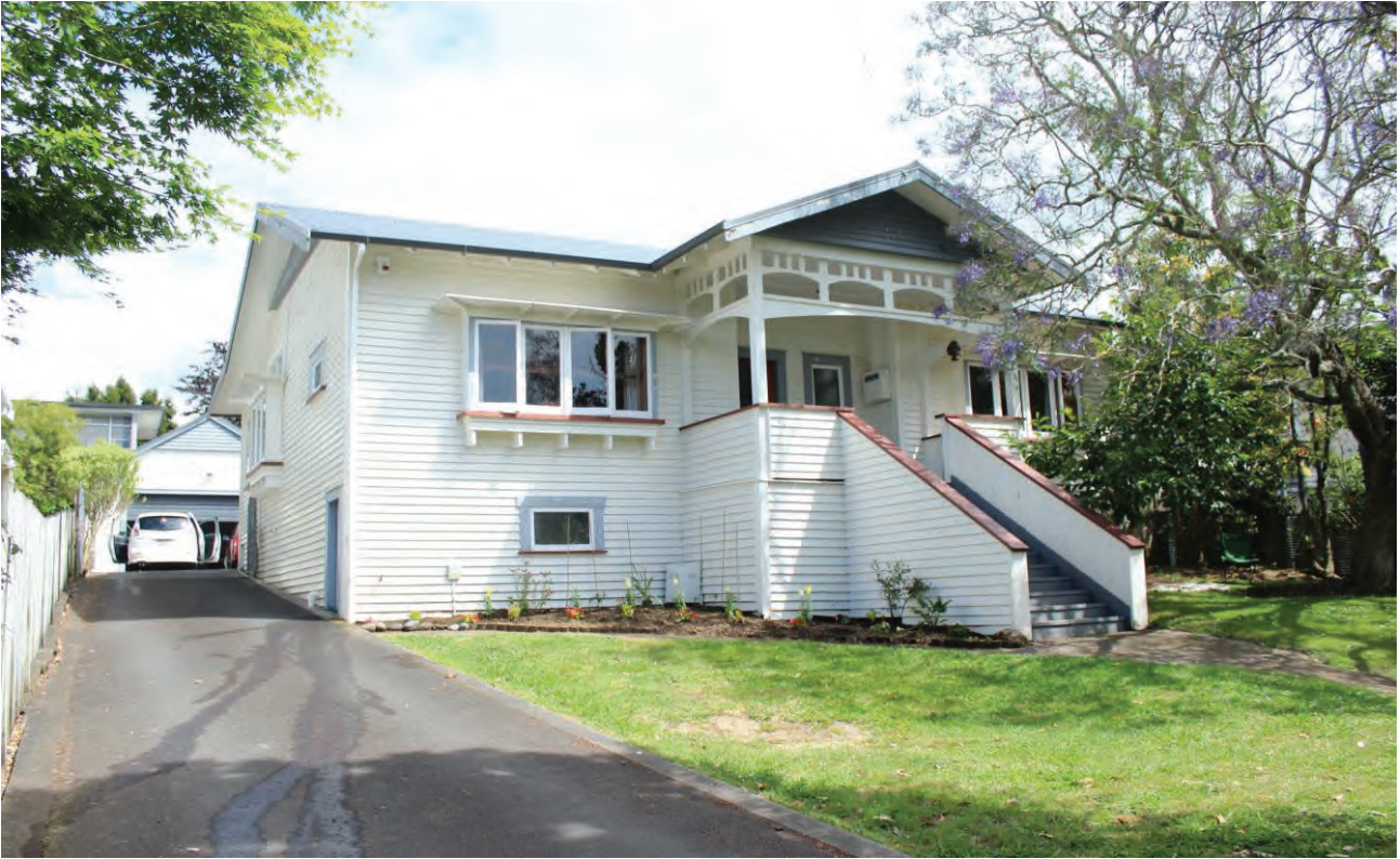
Figure 1: The dwelling at 27 Palmerston Street.
