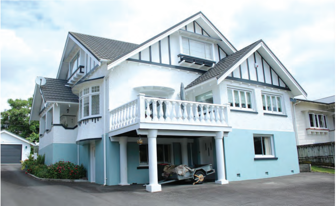
Figure 1: The dwelling at 25 Palmerston Street.
