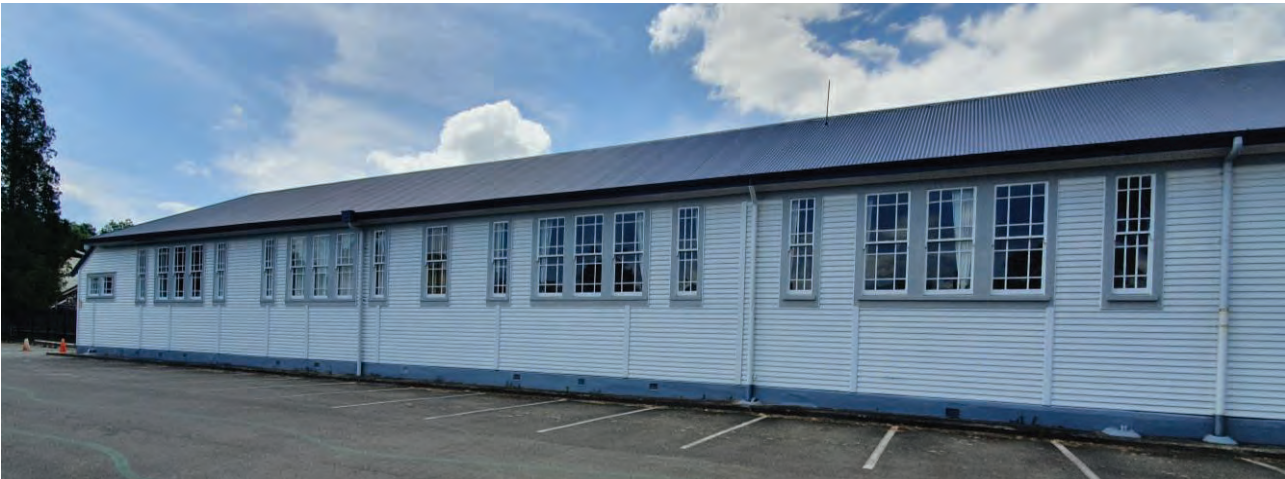
Figure 10: Part of the southern side of Hamilton West School today.
