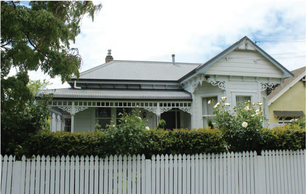
Figure 1: Villa at 54A Firth Street, 2021.
