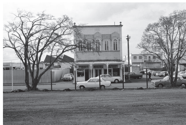
Figure 10: The building during operation as the St Vincent De Paul Hostel and Opportunity Shop, c.1970's. Source: ATL
