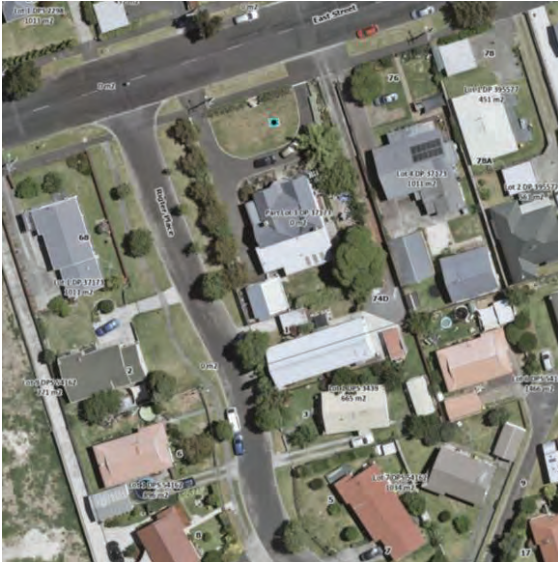
Figure 7: Aerial showing 74 East Street on a prominent street front. Source: HCC GIS Maps
