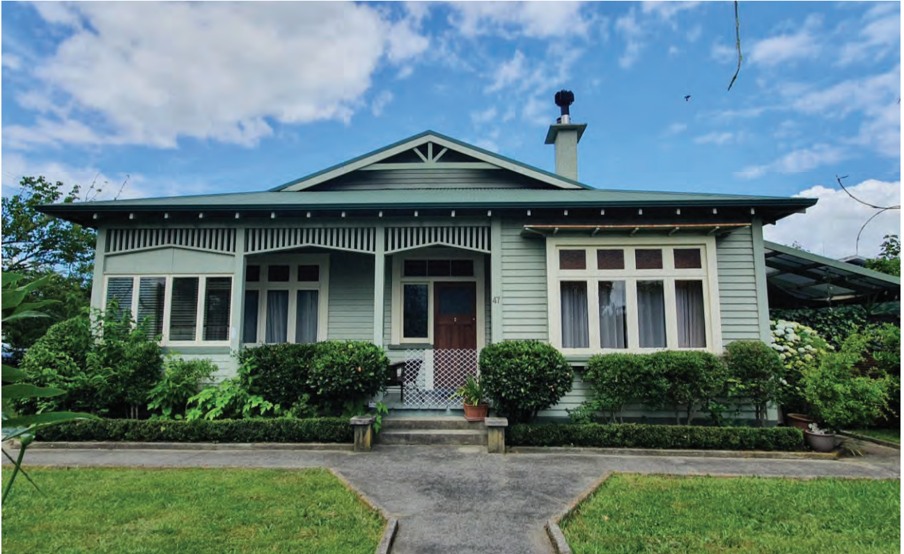
Figure 1: The dwelling at 47 Norton Road.
