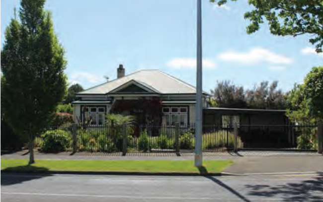
Figure 4: Street elevation of 106 Forest Lake Road showing the carport addition.
