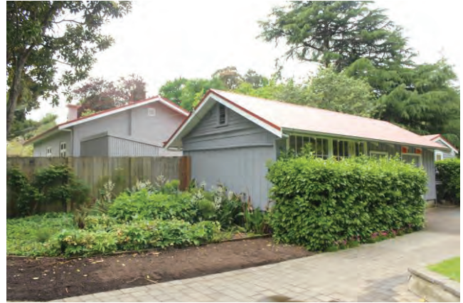
Figure 13: Garage built to the rear of the main dwelling.
