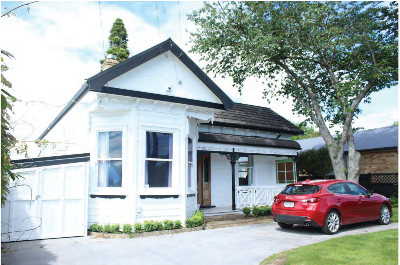
Figure 1: Villa at 60 Naylor Street.
