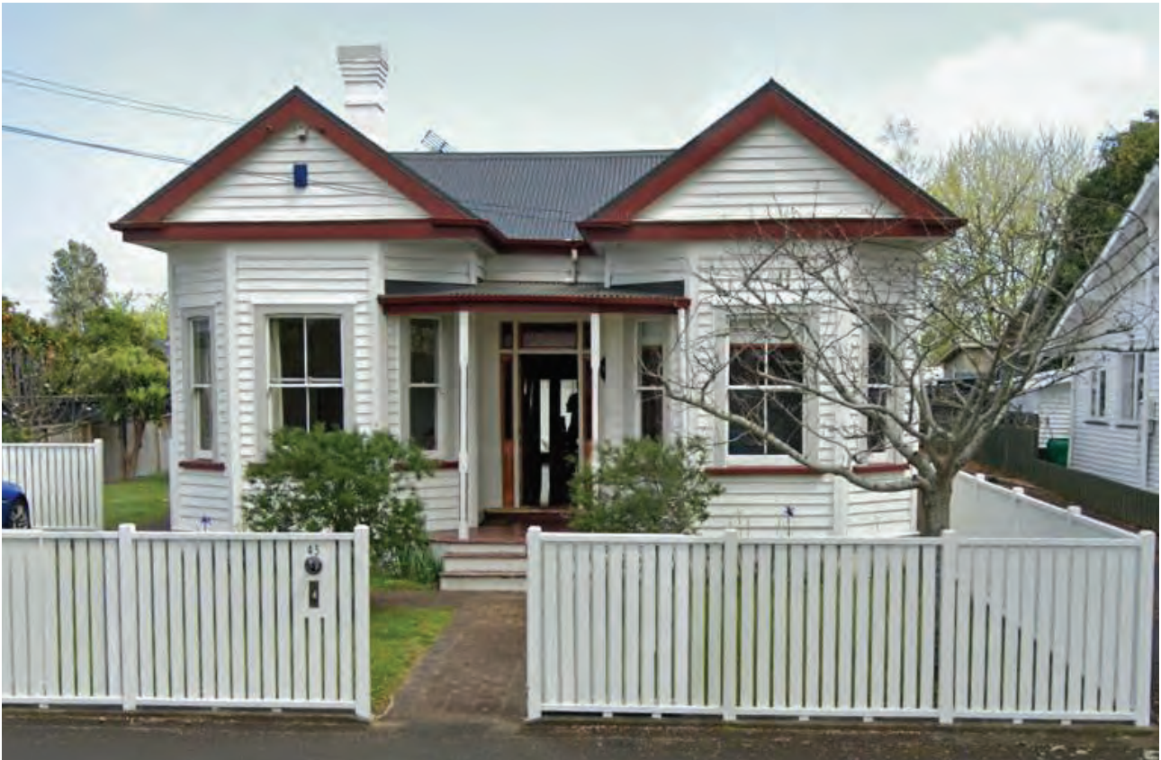
Figure 1: Double Bay villa at 45 Firth Street, 2021.
