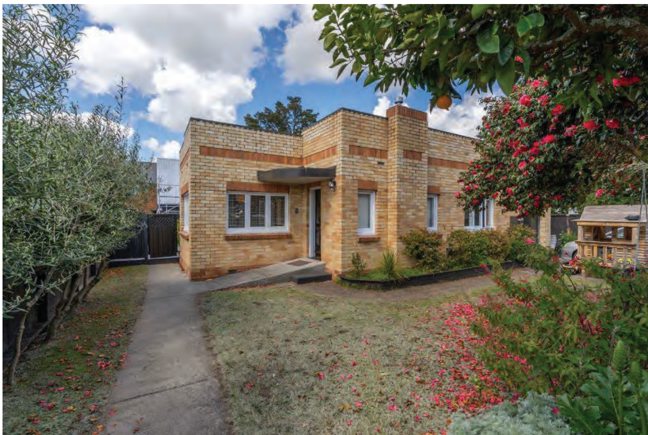
Figure 1: Art Deco styled residence in Huntly Brick.
