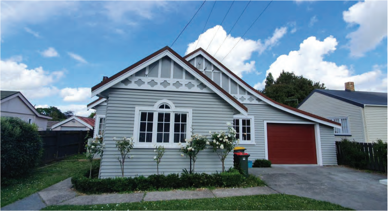
Figure 1: The property at 43 Horne Street.
