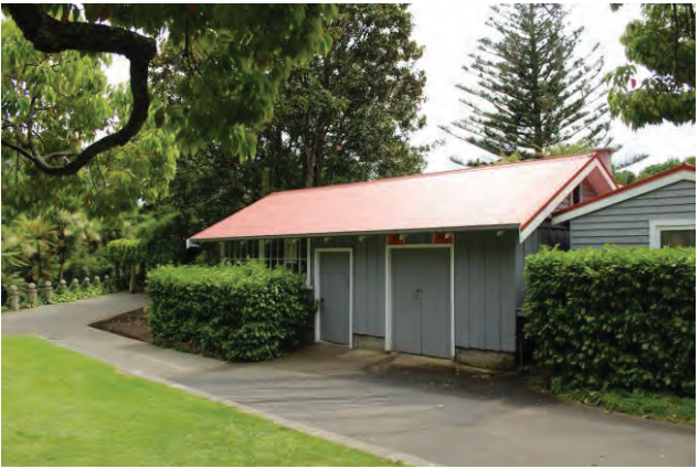
Figure 14: Garage built to the rear of the main dwelling.
