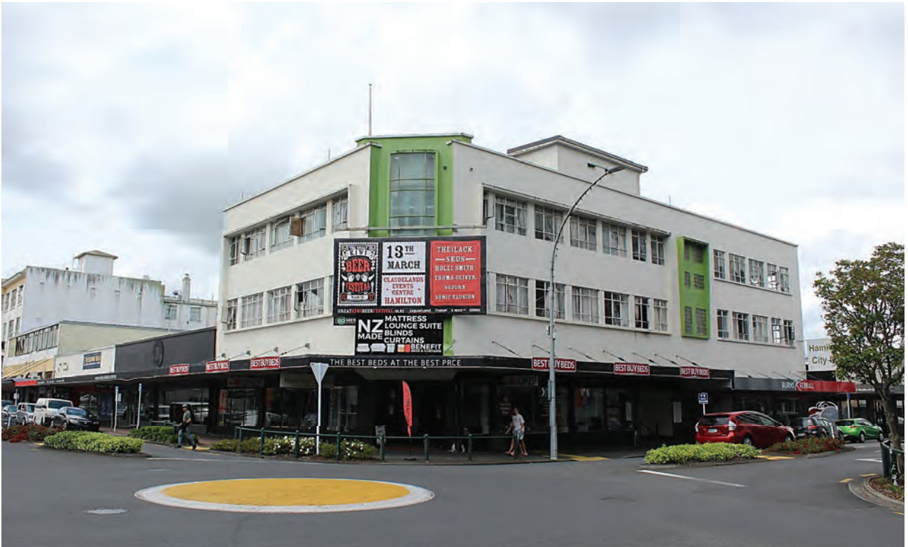
Figure 1: The former Farmers Building at 62 Alexandra Street.
