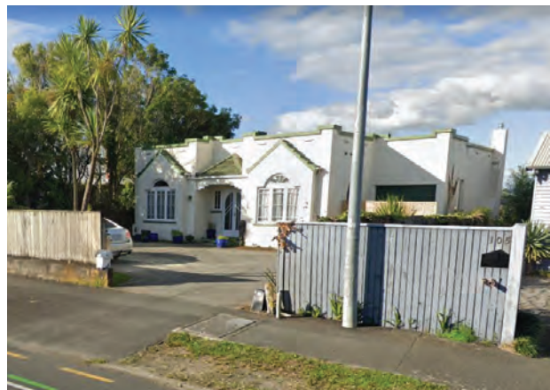
Figure 7: Aerial of 103 Pembroke Street in 2021. Source: Google Streetview
