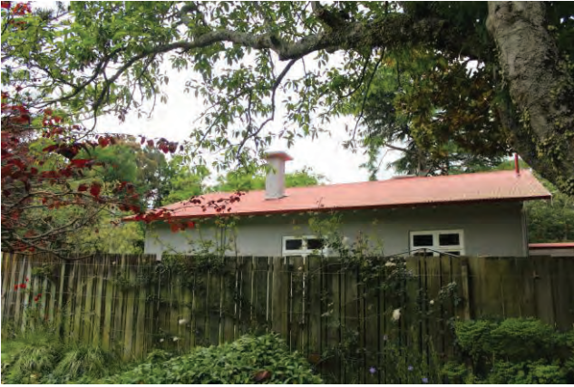
Figure 12: Side elevation of the building.
