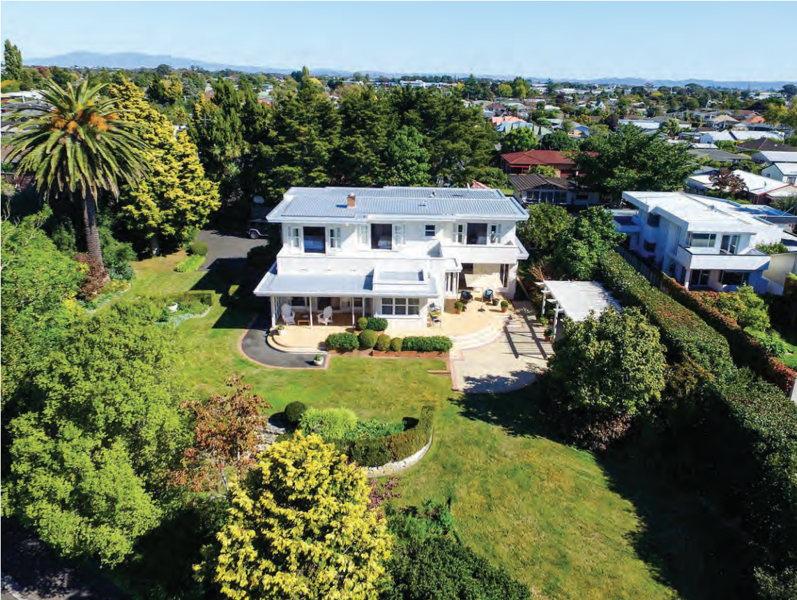
Figure 1: The dwelling at 65 Braid Road.
