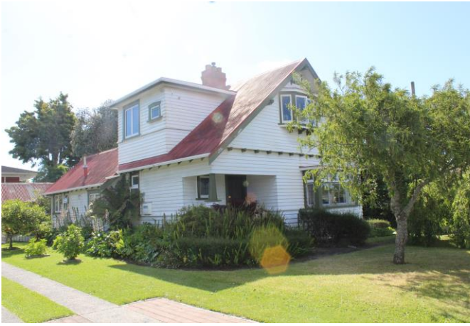
Figure 4: 409 Ulster Road, with large dormer additions to the roof.
