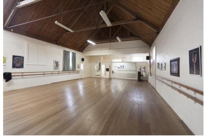
Figure 5: Interior of the building, showing an exposed truss roof and sarking. Source: Limelight Dance Academy
