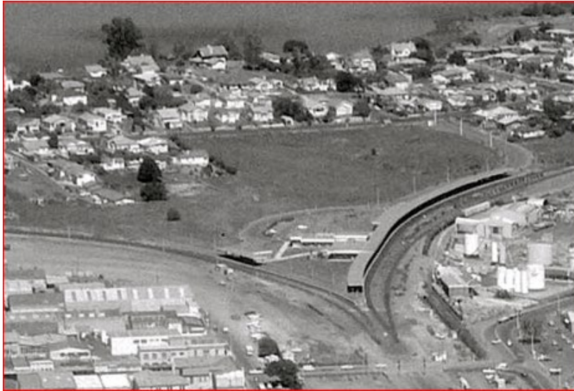
The new Hamilton Station in 1980, looking south with entrance off Queens Avenue in distance.
