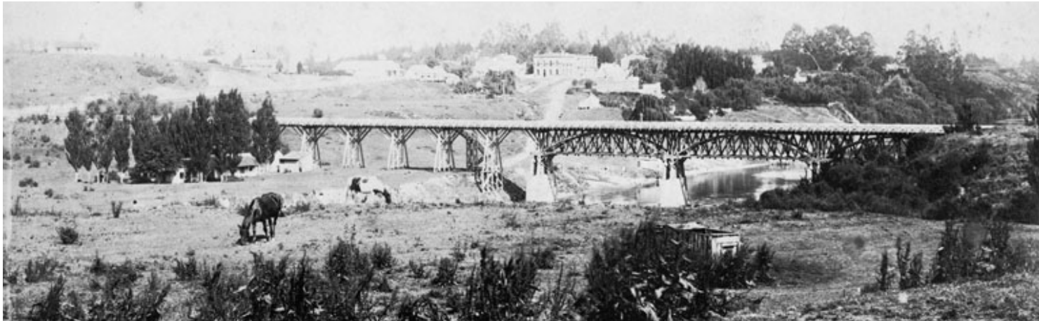
Below: Photography of the timber Union Bridge built in 1877 and joined West and East Hamilton until 1908 when it was replaced by the current Victoria Bridge. (HCL_00372)
