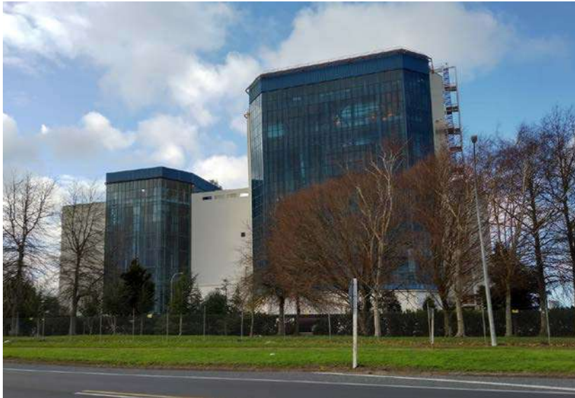
Fonterra from Te Rapa in 2023 showing glazed curtain walling.
