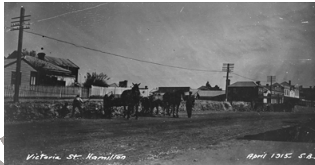
Figure 5.22 Workmen lowering the level of Victoria Street just south of Knox Street, April 1915, using picks and shovels. HCL_02792.
