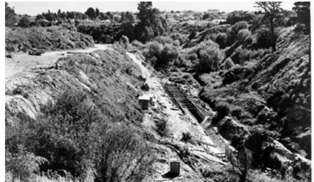
Figure 5.33. The beginnings of the construction of a culvert to channel the Waitewhiriwhiri Stream to allow the formation of the Ulster Street extension, c.1958-59. Photographer: A.E. Graham. HCL_04703.
