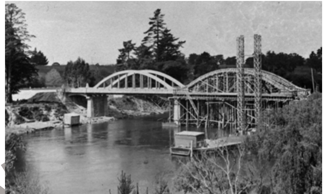
Figure 5.41. Fairfield Bridge under construction, with one of Roose's barges on the river, c. 1936. HCL_01006.
