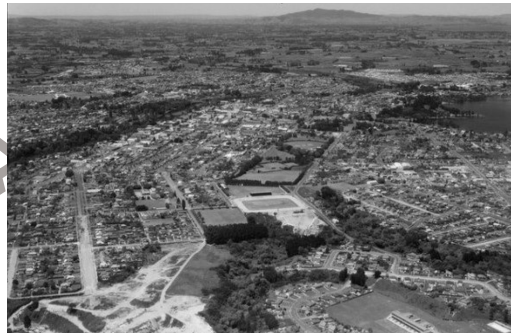
Figure 5.35. A view looking south across part of Maeroa and the Waitewhiriwhiri Stream, prior to the extension of Ulster Street (seen as a wide white strip running away from lower left) across the gully to join up with Gurnell Street. Earthworks related to the in-filling of the gully by deposition of spoil from Garden Place Hill are evident in the lower left of the photo in the vicinity of Whatanoa Pa. Whites Aviation, Alexander Turnbull Library. 12 Nov 1959 WA-51685.
