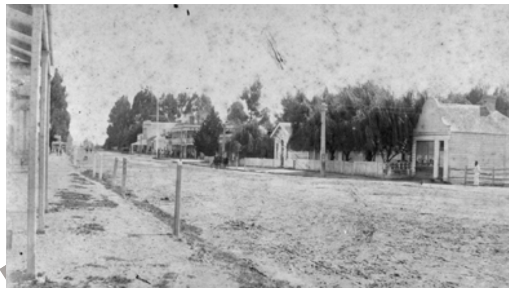
Figure 5.18. Looking north along Victoria Street from the vicinity of Knox Street, 1880s. The man in white (centre right) would be standing at the top of Grantham Street; the post office residence is behind the white picket fence and in the mid-ground further up the street is the Hamilton Hotel. There is a wide footpath on each side of the unsealed road and the eastern side has a formed gutter channel. Note all the hitching posts on each side of the road. HCL_02312.
