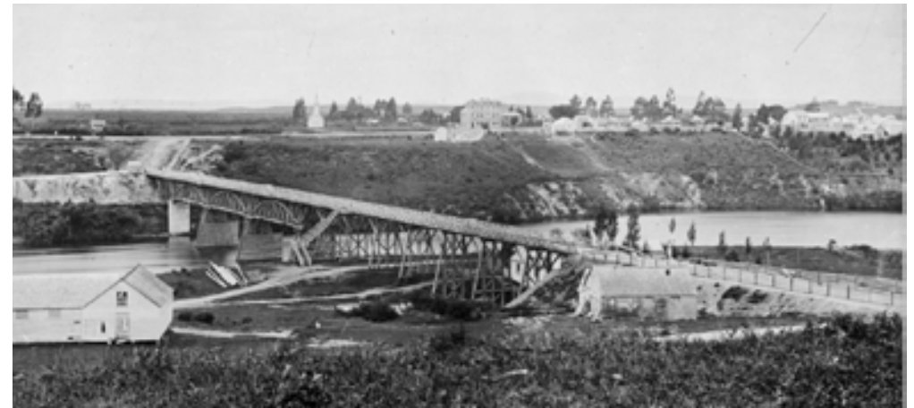
Figure 5.39. An early view of the Union Bridge looking from the west to the east shows the embankment necessary to raise the road at the western end, as well as formation work at the eastern end. In the foreground (left) is the government stables, while the other building by the bridge is probably Robert Williamson's forge. HCL_02758.
