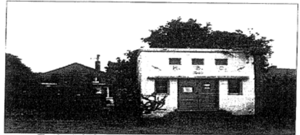
The electrical sub station in Galway Reserve dates from 1940.
