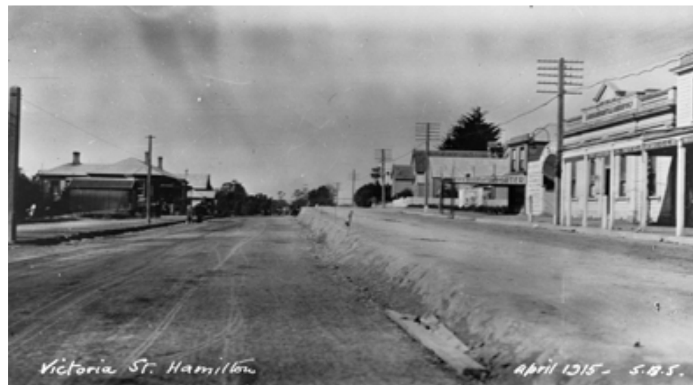
Figure 5.23 Workmen lowering the level of Victoria Street April 1915. Looking south from about Hood Street. HCL_02773.
