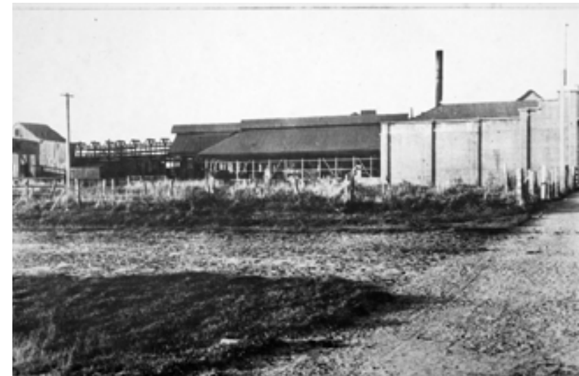
Figure 8.11. The northern aspect of the bacon factory. HCL_02328a.
