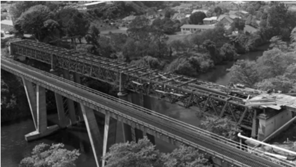
Figure 5.43 Claudelands Road Bridge being built, converted from the old railway bridge, with the new railway bridge beside it, 1967. Photographer A.E. Graham. HCL_02994.
