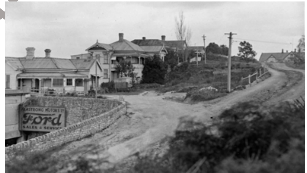
Figure 5.28. The access road to houses on Garden Place Hill was unsealed, apparently not even metalled, and steep. The roof of Hamilton West School is visible at top right, and the access road to Armstrong Motors is below the excavated scarp on the left. HCL_02780.
