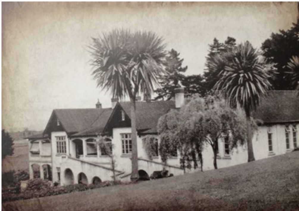
Figure 6.16 Old Men's Ward c. 1918. Collection of Waikato District Health Board.
