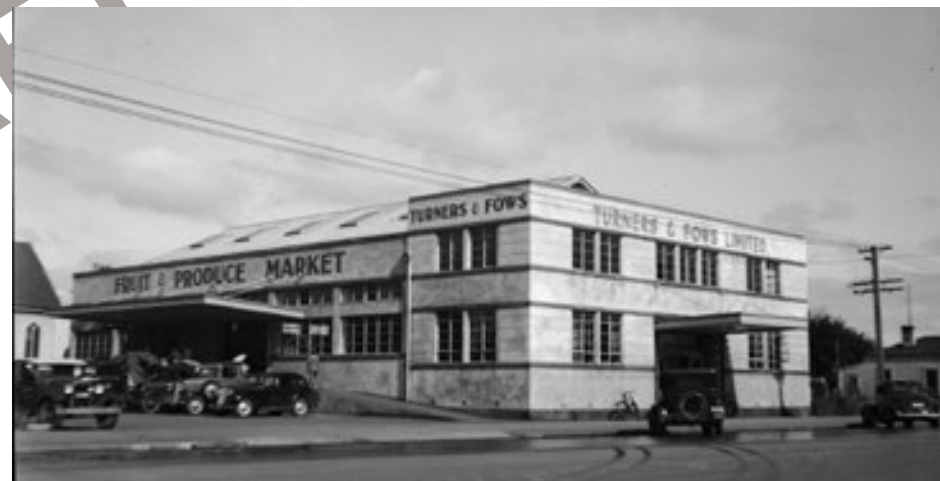
Figure 9.20 The purpose-built headquarters for Turners & Fows Ltd c. 1939.
