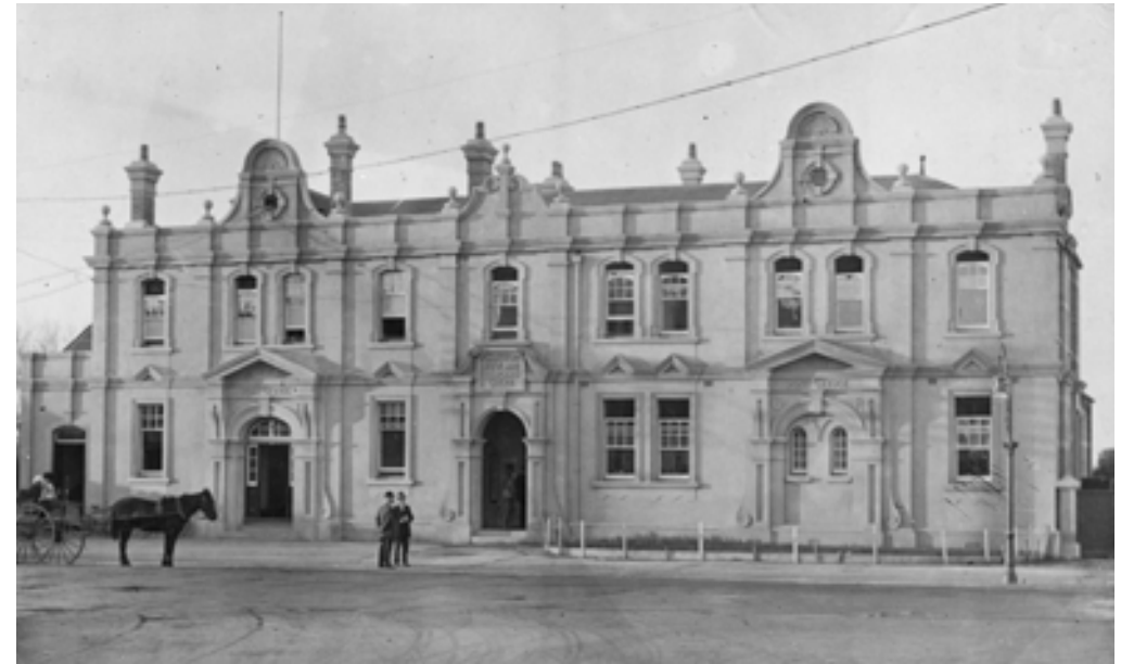
Figure 5.65 A c.1920 view of the post office after its extensive addition in 1916; the brickwork has been plastered. George Cartwright postcard. HCL_01405.
