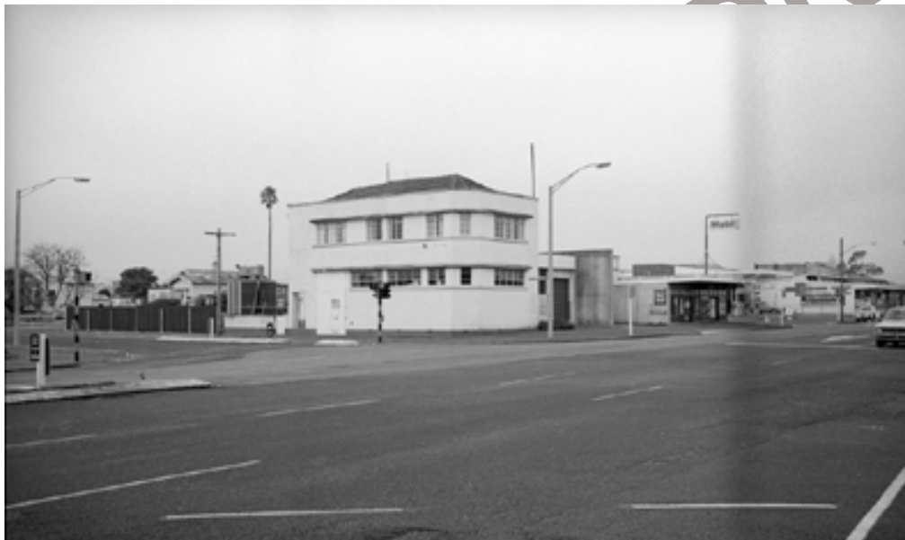
Figure 6.12 Claudelands Road electricity substation (formerly No.1 Substation), corner of Claudelands Road and Grey Street. HCL_M00277.34
