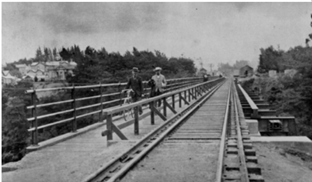
Figure 5.38. The newly-opened footbridge beside the railway bridge, 1908. HCL_02760.
