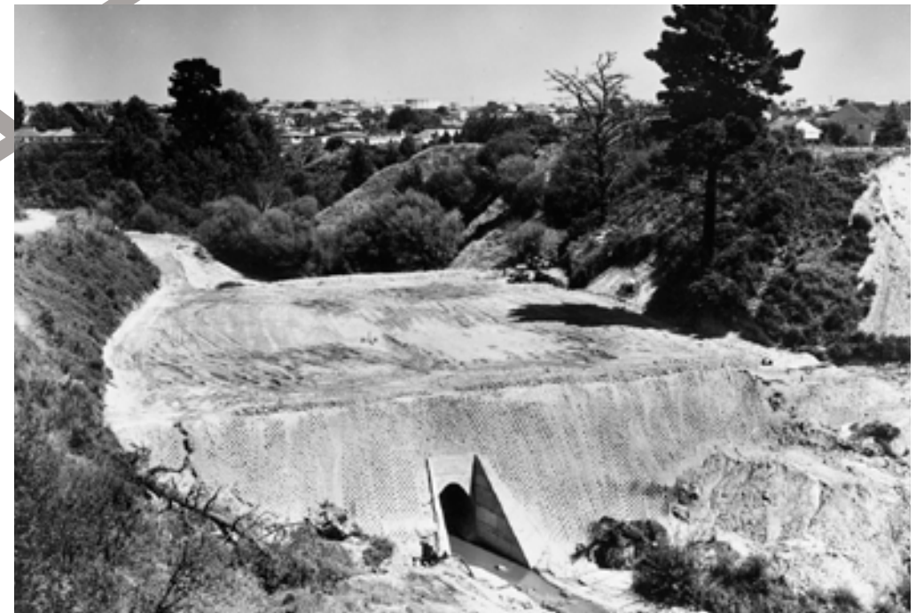
Figure 1.11 - Some of the culvert and road construction has been large-scale, such as the channelling of the Waitewhirwhiri Stream to enable the extension of Ulster Street, as seen in this 1960s photograph. Ulster Street then connected with Gurnell Avenue (far right upper). Photographer A.E. Graham. HCL_04707.
