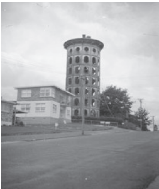
Figure 4.85 Tower Court flats were built in 1965. HCL_ M00401.3.
