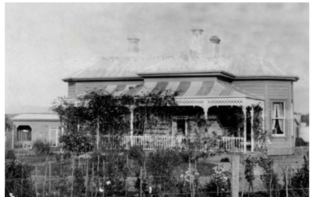
Figure 6.17 The front elevation of the medical superintendent's house in 1898. The bay window of the dining room is at right, with corrugated iron tanks beside the gardener's room-washhouse visible at far right. A gig and stable building is visible at back left. Collection of Waikato District Health Board.
