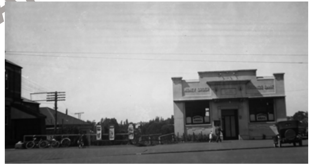
Figure 5.66 The Money Order and Savings Bank, built c.1920 as an adjunct to the post office (just visible at left). The building was later gifted to the Hamilton Borough Council by Helen Shaw Bell for use as an art gallery. HCL_01084.
