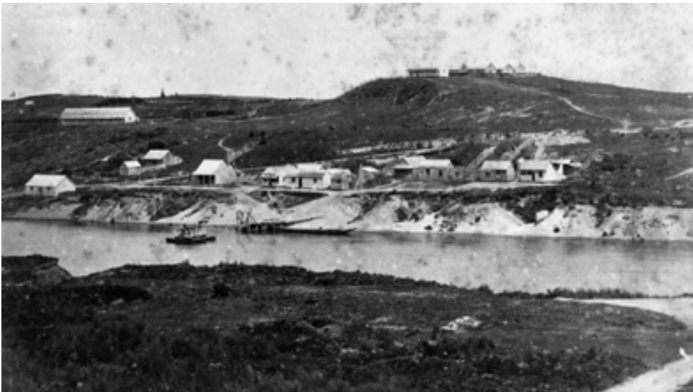
Figure 3.4. The earliest known photograph of Hamilton West, taken c. 1866, shows the Ferrybank landing with Commissariat buildings plus some unauthorised squatters' shops and houses, and the jetty for unloading supplies. On the hill above is Hamilton West redoubt with four buildings within a ditch and bank defensive structure and another building outside the bank. At left is the militia hospital, on the site of the current police station. The punt, made up of two small canoes tied together with a platform, is shown crossing the river, while a long canoe is tied to the jetty. HCL_003175.
