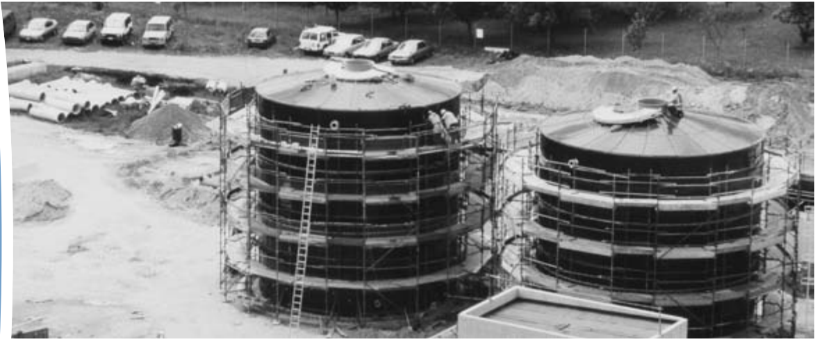
The new digester buildings under construction at the Wastewater Treatment Plant.
