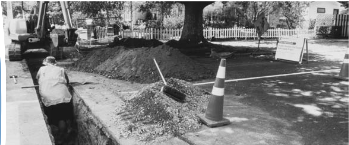
Water supply pipes on Norton Road being replaced with new long-lasting PVC pipes.
