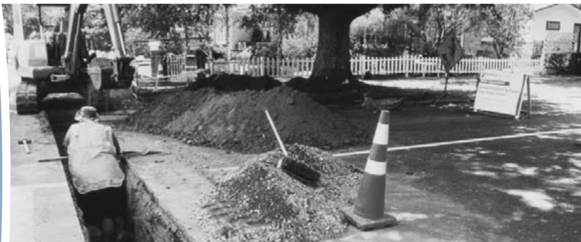
Water supply pipes on Norton Road being replaced with new long-lasting PVC pipes.
