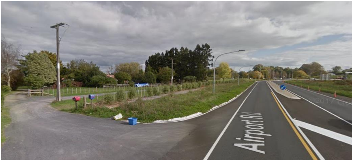
Figure 26 Example of reduced height street lighting on Airport Road, Hamilton.
