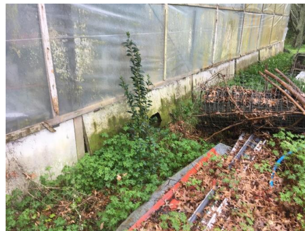
Photograph 54: Asbestos cladding on shed - 361 Peacockes Road
