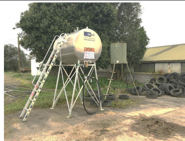
Photograph 32: New and old diesel AST adjacent to old milking shed
