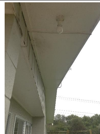
Photograph 44: Potential asbestos on dwelling at 461 Peacockes Road
