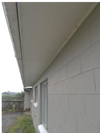
Photograph 45: Potential asbestos on dwelling at 461 Peacockes Road
