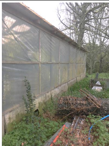
Photograph 55: Asbestos cladding on shed and surrounding stockpiled materials - 361 Peacockes Road
