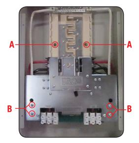
**3)** Remove mechanism from cabinet and turn upside down to expose fuses and replace fuse as necessary
