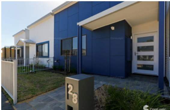
Hardieplank Construction (Source: Corelogic)
