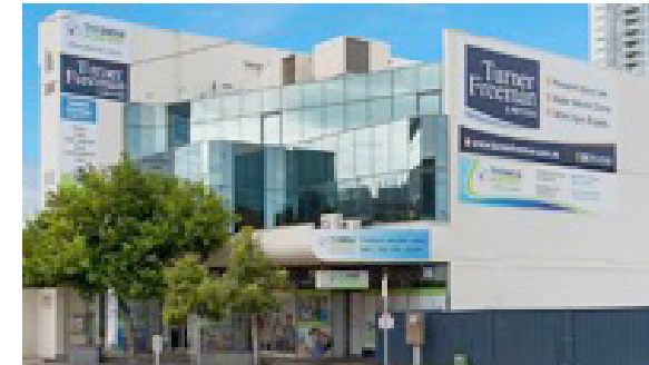
56 Nerang St, Southport - sold April 2018, $6.973M, AY 6.71%, Rate $3,467/m 2 NLA (Source: www.commercialrealestate.com.au )
