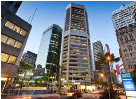
300 Queen Street, Brisbane (Source: www.realcommercial.com.au )
