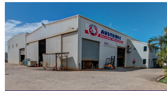
12-16 Progress Drive, Mackay
