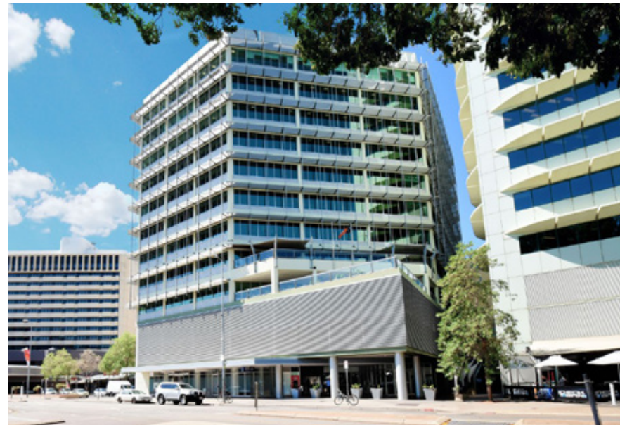
TIO Building, 24 Mitchell Street Darwin (Source: www.realcommercial.com.au )
