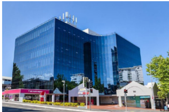
90 Crown Street, Wollongong (Source: www.realcommercial.com.au )
