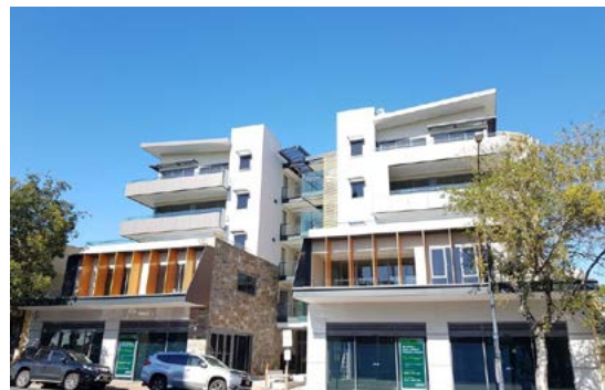
Retail tenancies for lease on the ground floor of the Nuova Apartments, Norwood. Source: Realcommercial
