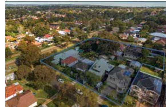
13-21 University Road & 1-5 Pinnacle Street Miranda (Source: www.realcommercial.com.au )
