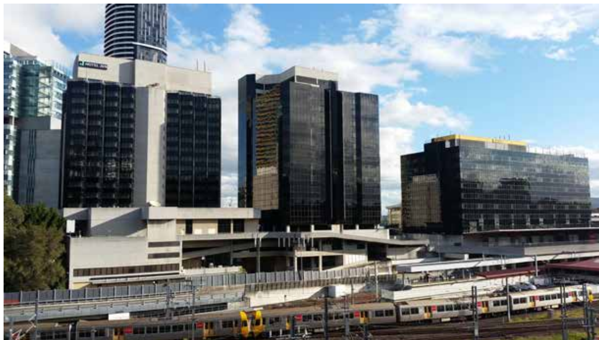
The Brisbane Transit Centre...To be demolished for the Cross River Rail Project (Source: ???)
