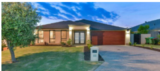
Beckingham Parkway, Baldvis
