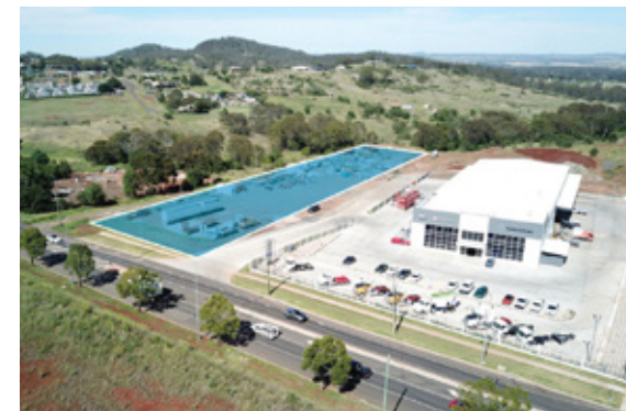
373 Anzac Avenue, Harristown (Source: www.commercialview.com.au )
