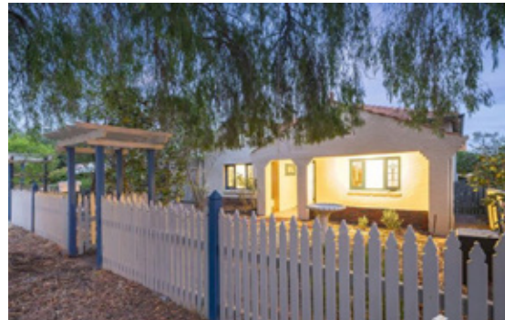
Figure 9 - Surrey Road, Rivervale Source: CoreLogic
