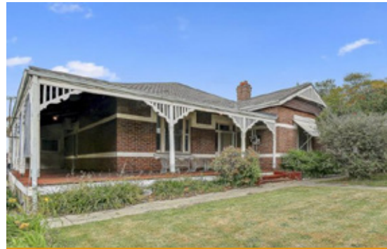
Figure 3 - Great Eastern Highway, Greenmount Source: CoreLogic
