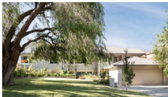
Facade at Athelstan Road, Cottesloe
