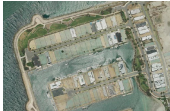
Current Development at Othello Quays, North Coogee Source: Department Of Planning, Lands & Heritage
