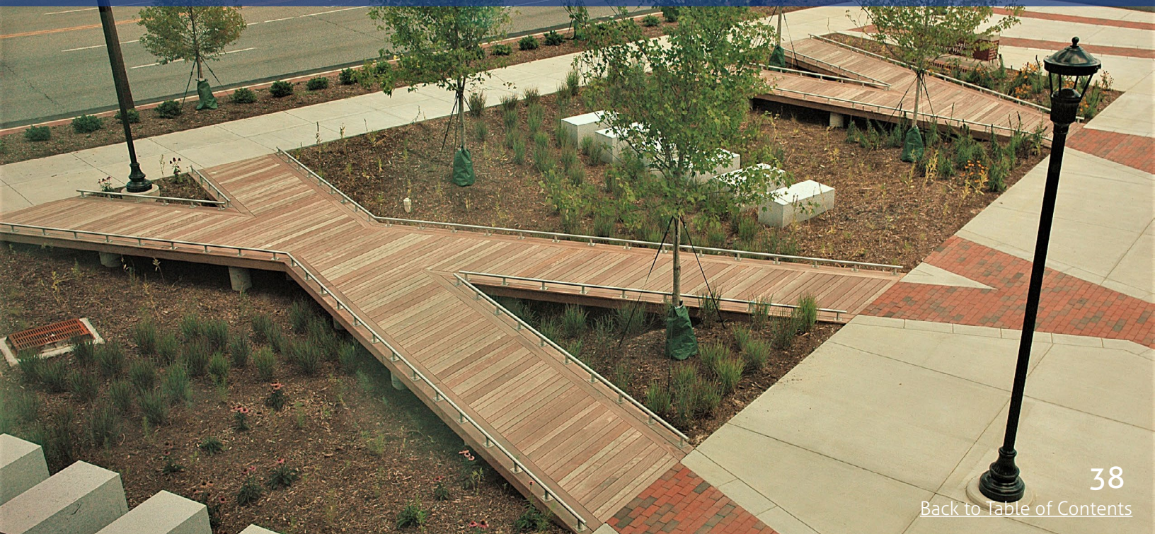
Bioswale stormwater biofiltration system at UNC Greensboro. Courtesy of University of North Carolina, Greensboro.
