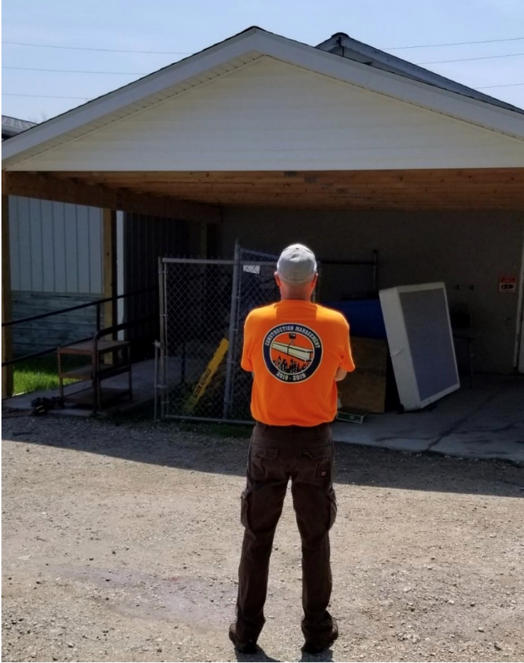
Photo Caption: Phyllis Zumkehr Portage County Clothing Center donation drop-off after finished shelter construction, protecting drop-off donations during off-hours from the elements.
