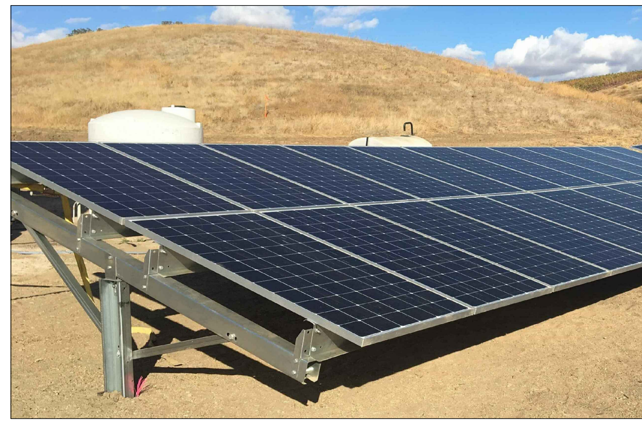
TYPICAL RBI RACKING ARRANGEMENT
