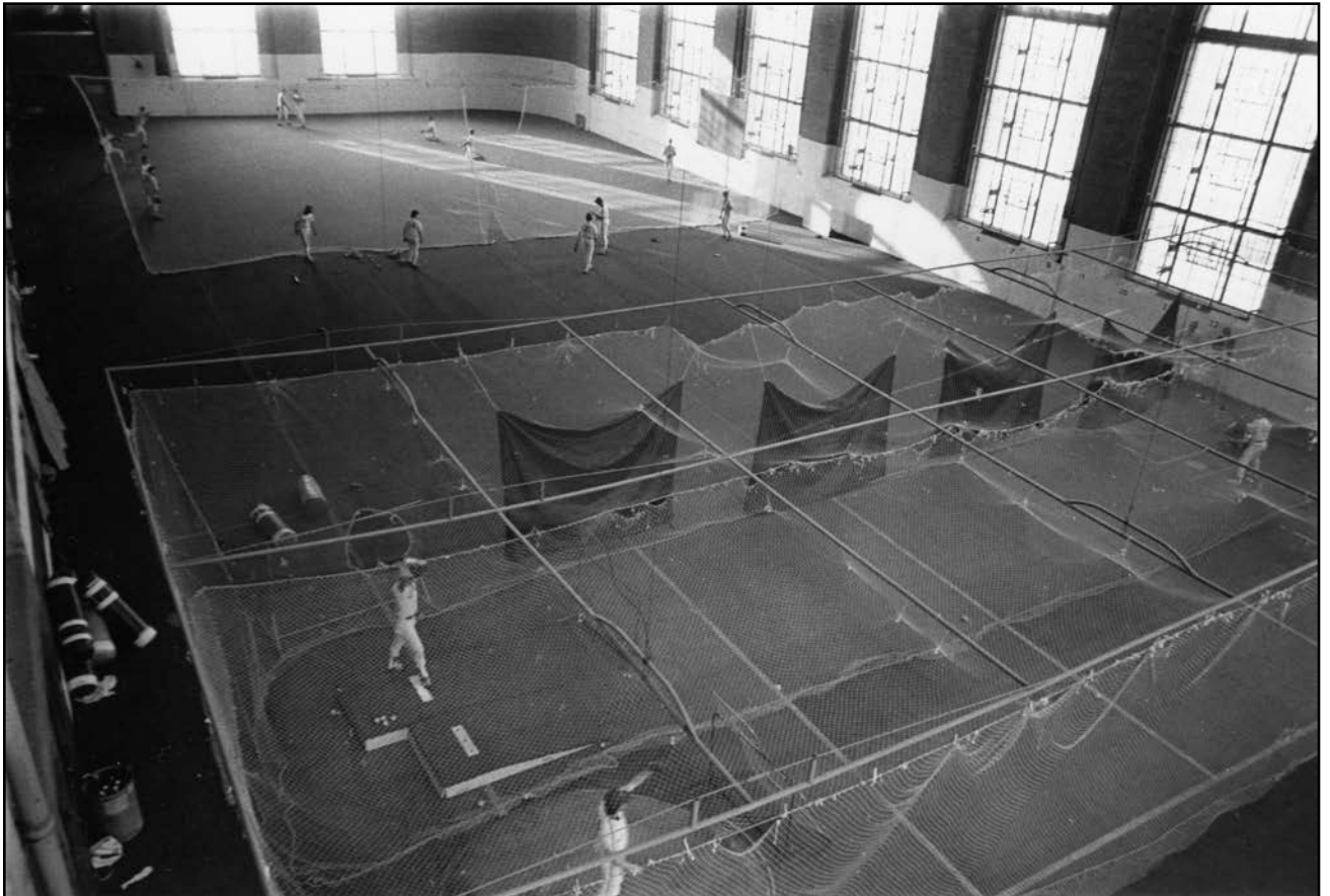
(Fig. 70.25) Nebraska Baseball shown practicing in Schulte Fieldhouse. The nets were raised for other sports. The Suh Strength Complex later occupied this exact footprint as Schulte was torn down and rebuilt.
