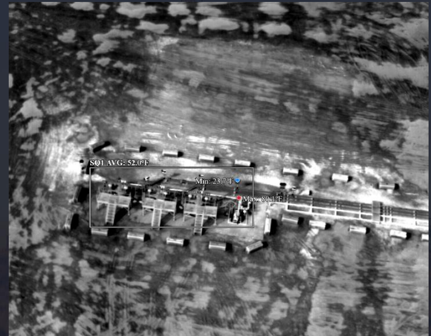
Thermal Drone Surveys
