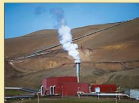
Fig. 20 Geothermal energy provides economic benefits.
